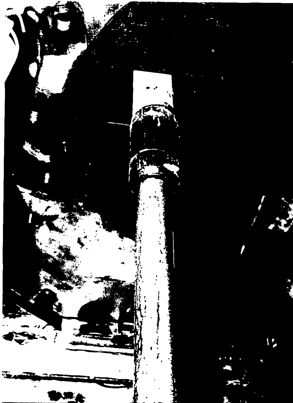
Figure 4a. Center thermowell - Inconel 690 collar below alumina insulator (WSRC-FM-95-0049-90).
