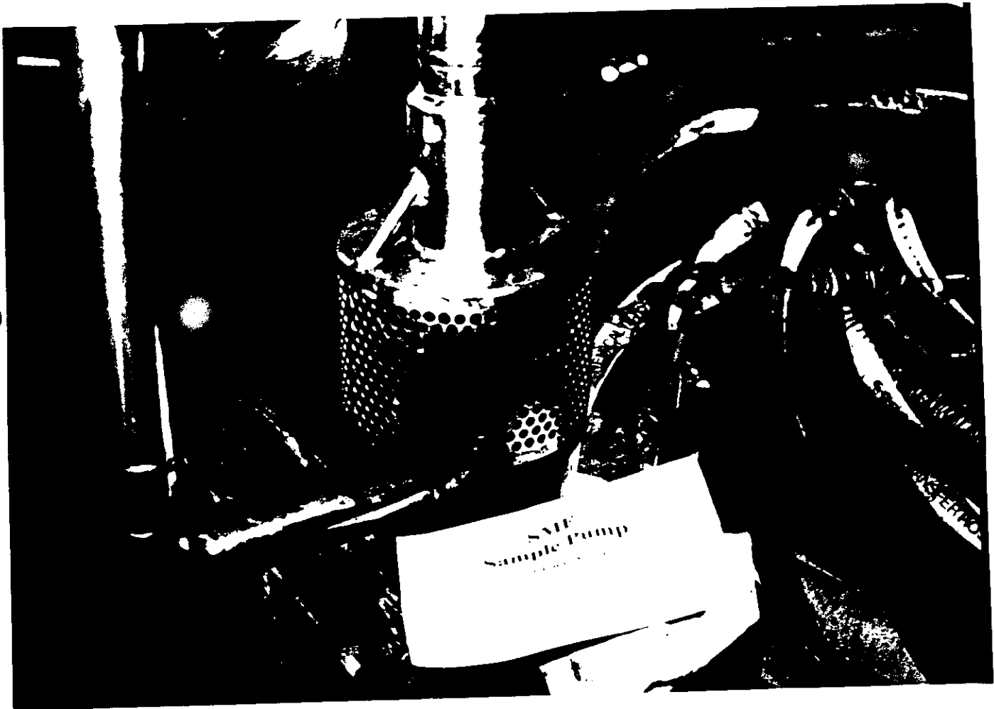
Figure 11. Photograph of the strainer and suction line from the SME sample pump (WSRC-FM-95-0006-8). Note welds and strainer show visible signs of significant erosion.
