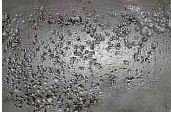
Figure 7. Pitting corrosion on carbon steel [39]. Note that this is not pitting from the SRS waste transfer line system.
