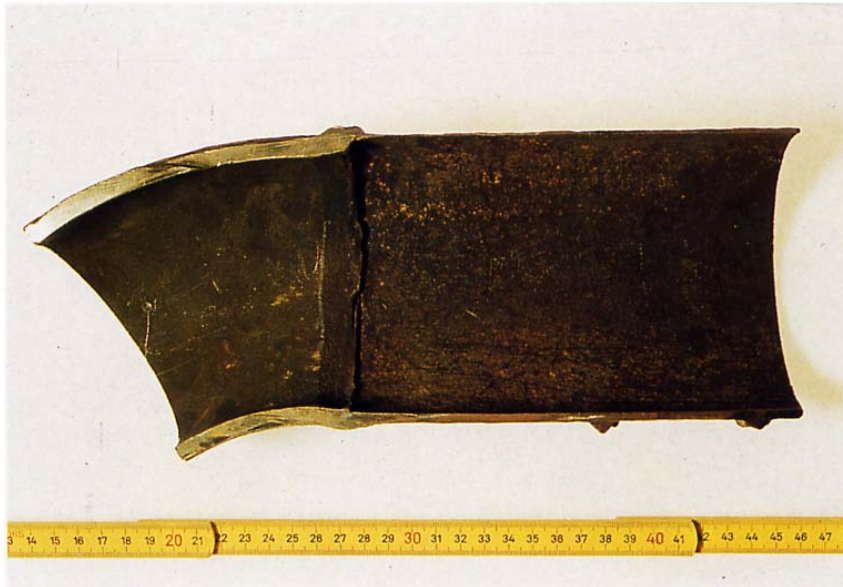
Figure 4. Straight Section of Pipe Exhibiting General Corrosion of Carbon Steel [39]. Note that this is not piping from the SRS waste transfer line system.
