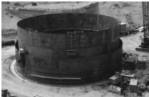
Figure 4-11. Secondary Liner Wall Fabrication and Primary Tank Wall (Photo 68847-37) (Taken 4-18-75)
