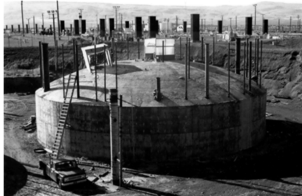
Figure 4-18. Completion of Tank Dome Concrete (Photo 70273) (Taken 10-22-75)
