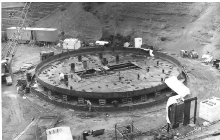
Figure 4-8. Crews Fabricating Primary Tank Bottom (Photo 66771-26) (Taken 11-21-74)
