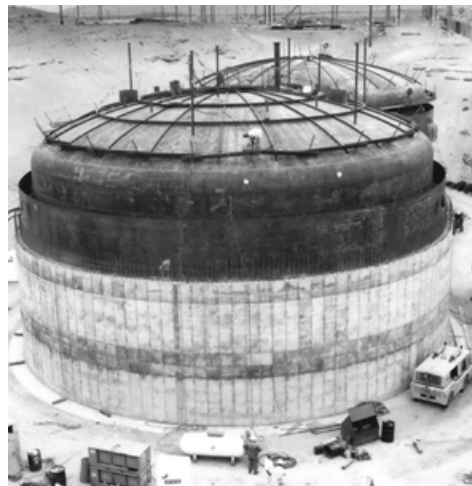
Figure 4-13. Two Courses of Concrete Have Been Poured (Photo 69402-38) (Taken 6-19-75)
