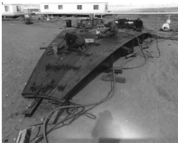
Figure 4-9. Fabricators Welding the Tank Dome Sub-Assemblies (Photo 67722-39) (Taken 3-20-75)
