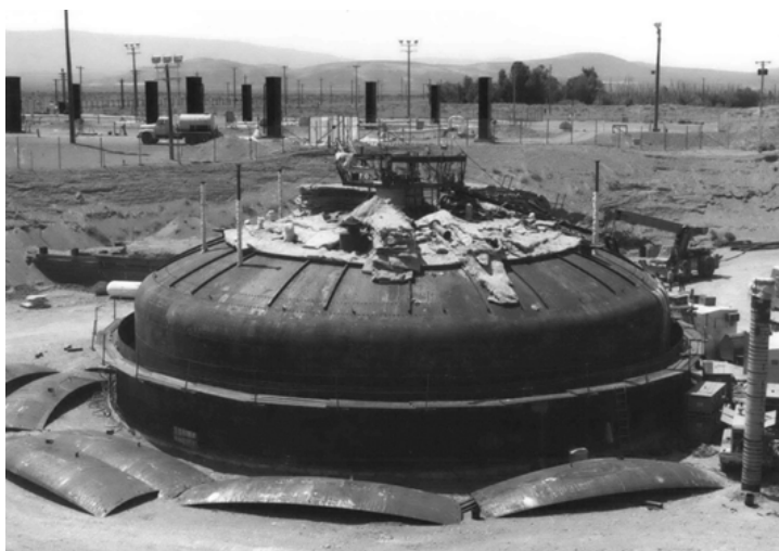
Figure 4-15. Partial Backfill of Tank SY-103 (Photo 69620-44) (Taken 7-22-75)
