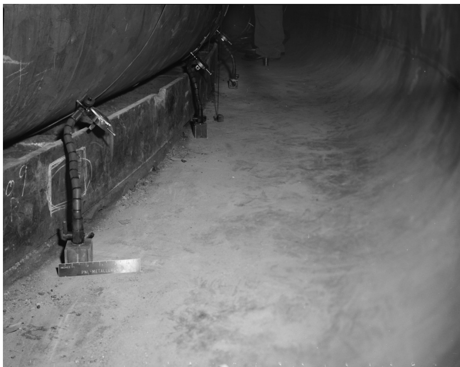
Figure 5-6. Battelle Strain Gauges on Primary Tank SY-103 (Photo 756534-20) (Taken 9-12-1975)
