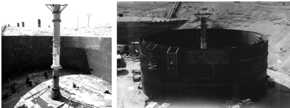
Figure 4-10. Tank Dome Support (Photo 68847-35 and 68847-38) (Taken 4/18/75)
