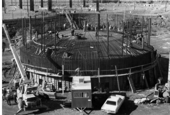
Figure 4-17. Crews Installing Rebar Prior to Concrete Dome Pour (Photo 70273-26) (Taken 10-22-75)
