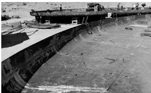
Figure 4-4. Secondary Liner Lower Knuckle Section for Tank 241-SY-101 (Photo 64516-8) (Taken 8-20-74)
