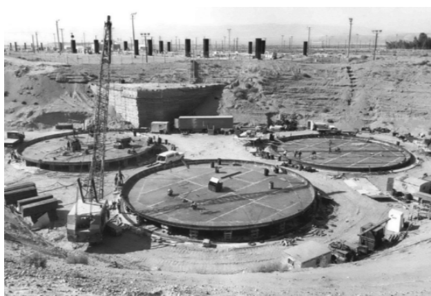
Figure 4-2. Crews Fabricating Secondary Liner Bottom (Photo 64775-12) (Taken 9-23-74)
