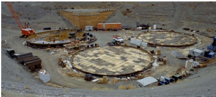
Figure 4-7. Protective Layer Installed Over Refractory for 241-SY-101 and 241-SY-102. (Photo 66534-1) (Taken 10-21-74)
