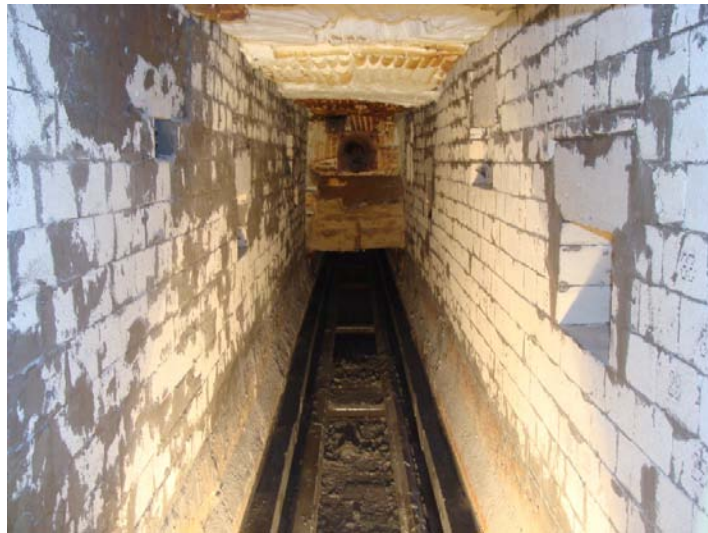
Figure 4: Refractory Reline in Zones 2-3 of the LHF
