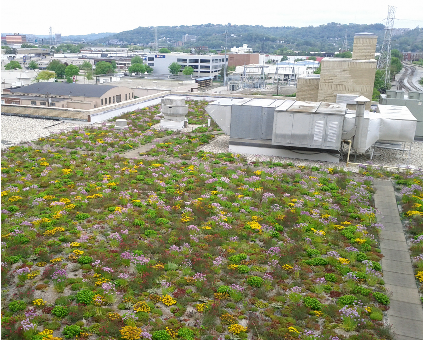
GREEN ROOF INSTALLED AS PART OF PROJECT 1 [2011]
