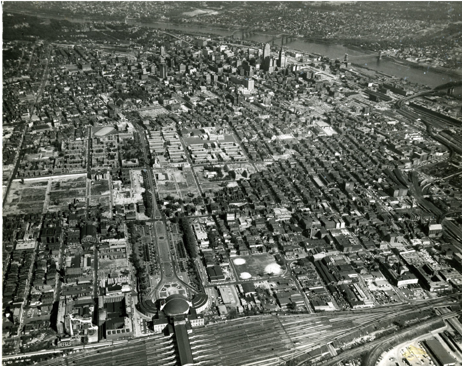
1950S, LAUREL HOMES, LINCOLN COURT, AND RICHMOND VILLAGE WERE CONSTRUCTED TO THE EAST, DRAMATICALLY CHANGING THE WEST END COMMUNITY.
