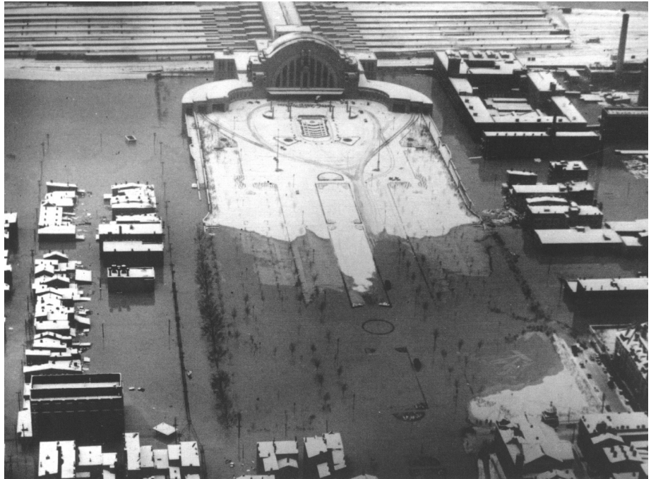
THE TERMINAL WAS DESIGNED TO REMAIN ABOVE THE FLOOD PLAIN, WHICH IT DID IN THIS IMAGE OF A 1937 FLOOD.
