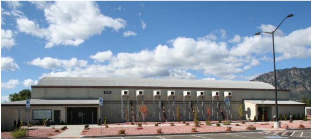
Figure 22. Event center exterior installation
