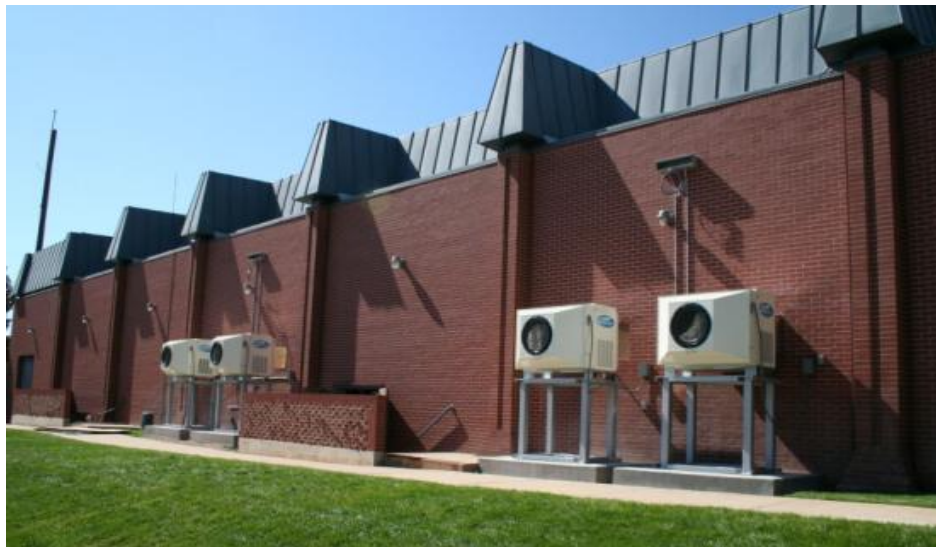
Figure 20. Theater exterior installation
