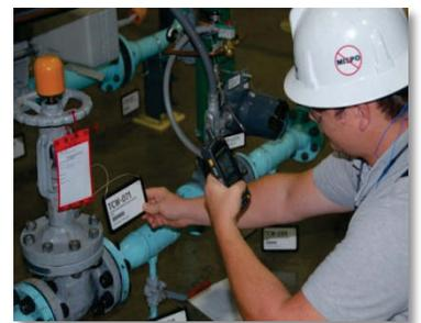
**Figure 5 Operator at Catawba Nuclear Station using hand-held technology for component identification**
