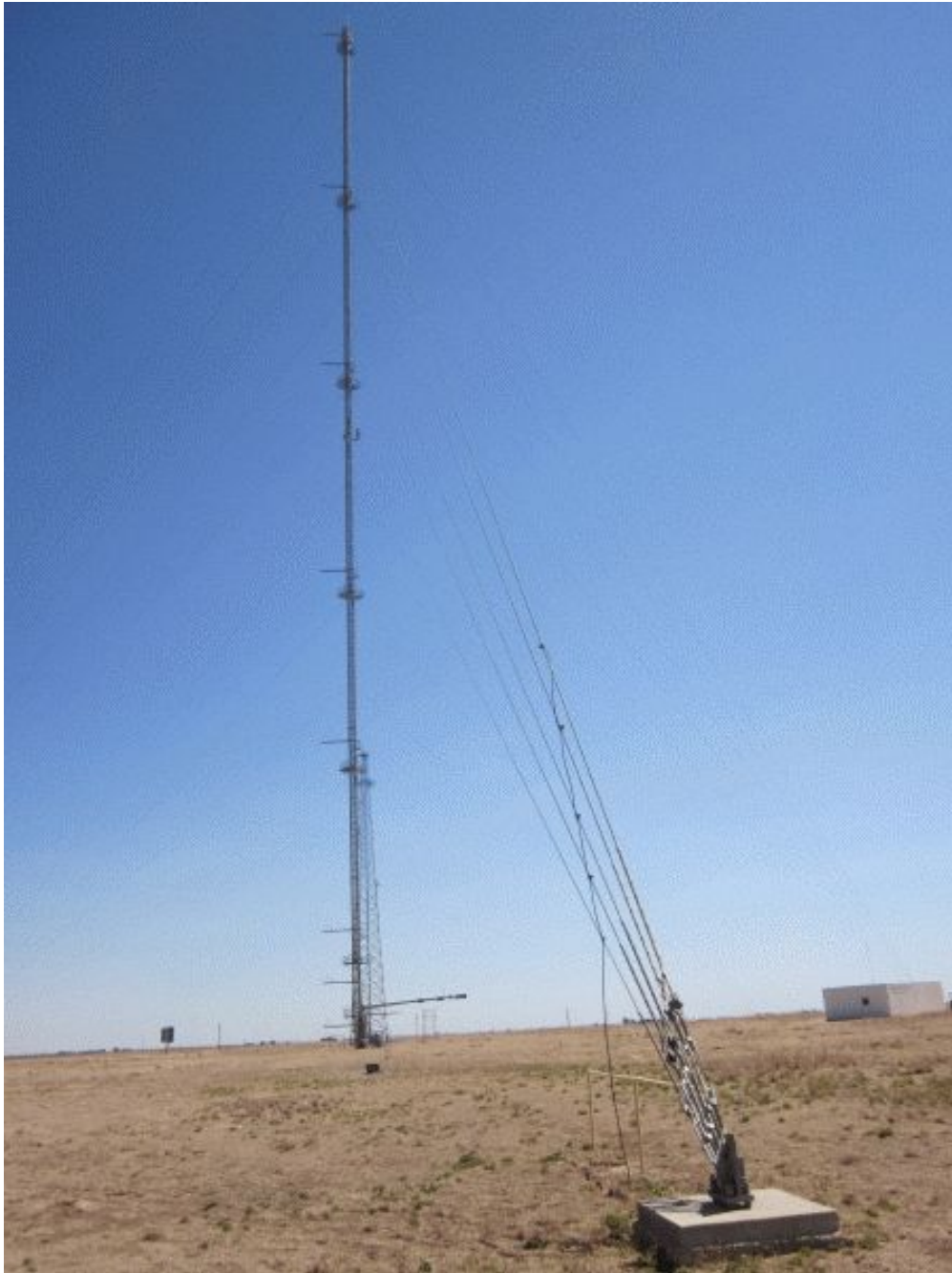
Fig. 3.31. The photo shows the entire 200 meter height of the meteorological tower at the Reese Technology Center. The tower includes measurements at 10 stations along its vertical extent.
