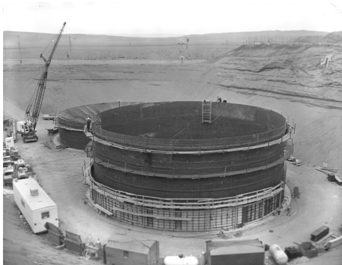
Figure 4-7. Tank AY-102 (foreground) Secondary Liner Wall Fabrication and Concrete Forms (Photo No. 8131) (Taken 3/27/1969)
