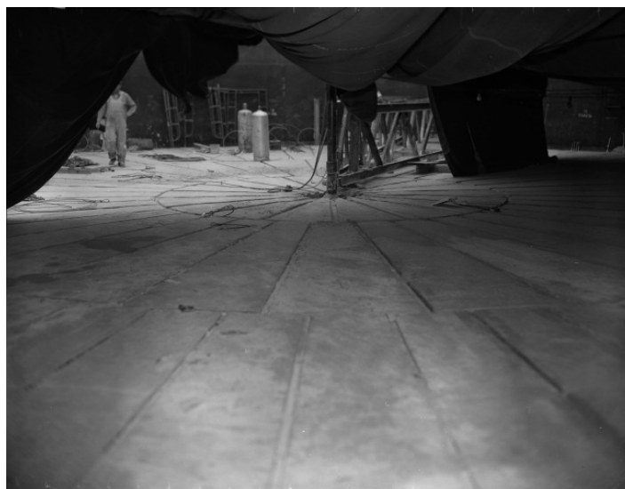
Figure 4-6. Completed Refractory in Tank AY-101 (Photo No. 8124) (Taken 3/27/1969)
