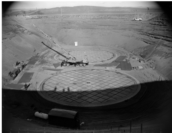
Figure 4-2. Foundations for Tank AY-101 (background) and Tank AY-102 (Photo No. 8041) (Taken 11/22/1968)
