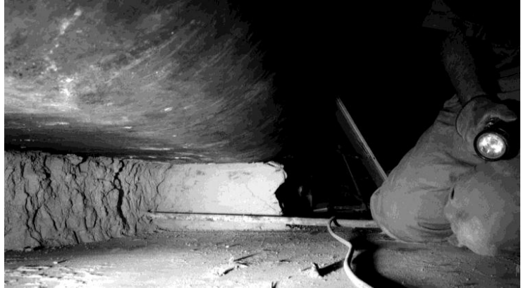
Figure 5-3. Tank AY-101 Refractory Repair
