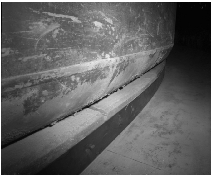
Figure 5-7. Tank AY-102 Finish Perimeter Concrete Support Ring
