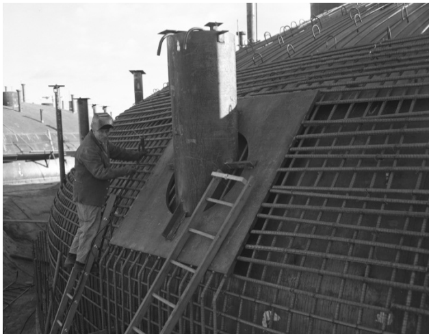
Figure 4-13. Fabricator Installing Rebar (Photo No. 51084-1) (Taken 11/17/1969)
