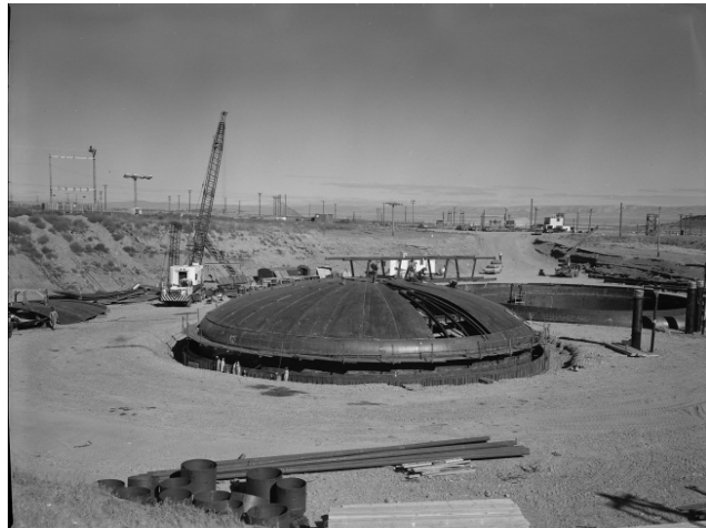
Figure 4-9. Tank AY-102 Primary Dome Construction (Photo No. 50449-1) (Taken 8/19/1969)
