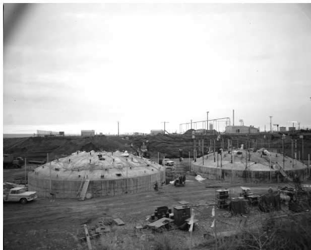
Figure 4-16. Concrete Dome Complete, Looking Southwest (Photo No. 51305-13) (Taken 12/22/1969)
