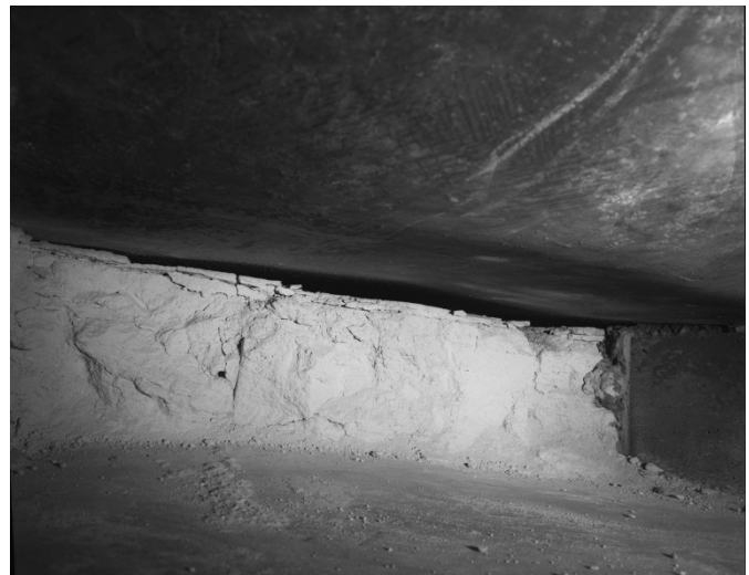
Figure 5-5. Tank AY-101 Refractory Repair (Photo No. 52788-8) (Taken 8/3/1970)
