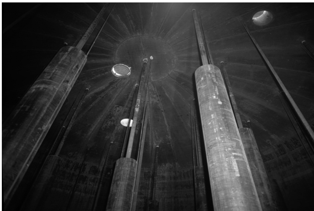
Figure 4-15. Center of Dome and Completed Internals of Tank AY-102 (Photo No. 51660-18) (Taken 2/20/1970)
