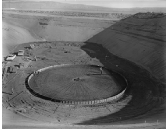
Figure 4-1. Laying Reinforcing Steel for Foundations (Photo No. 8000) (Taken 9/25/1968)
