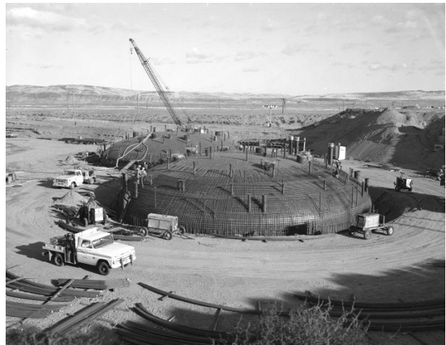
Figure 4-14. Rebar Installation for Concrete Dome Pour (Photo No. 51084-2) (Taken 11/17/1969)
