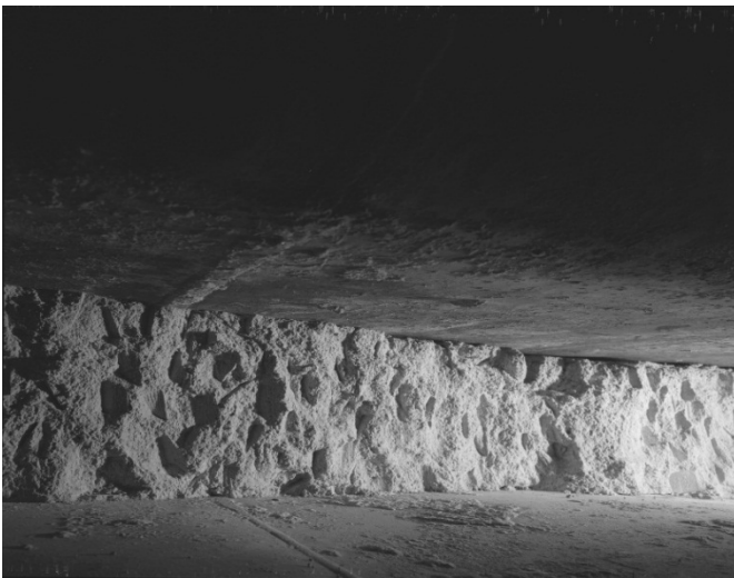
Figure 5-4. Tank AY-101 Refractory Repair (Photo No. 52720-3) (Taken 7/23/1970)
