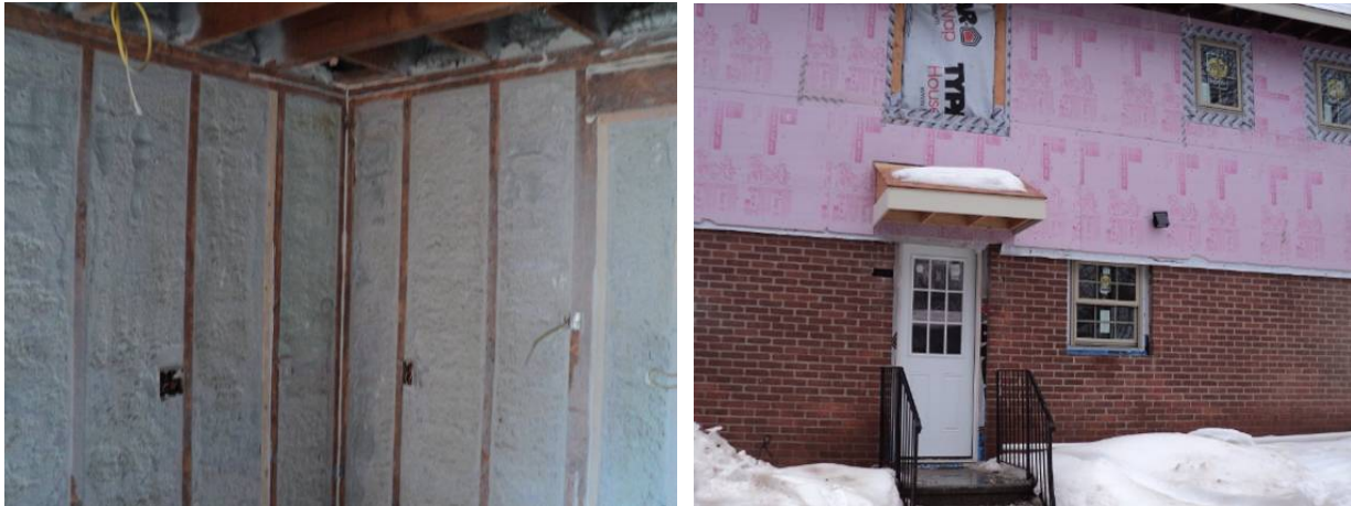
Figure 10. Above-grade walls after retrofit
