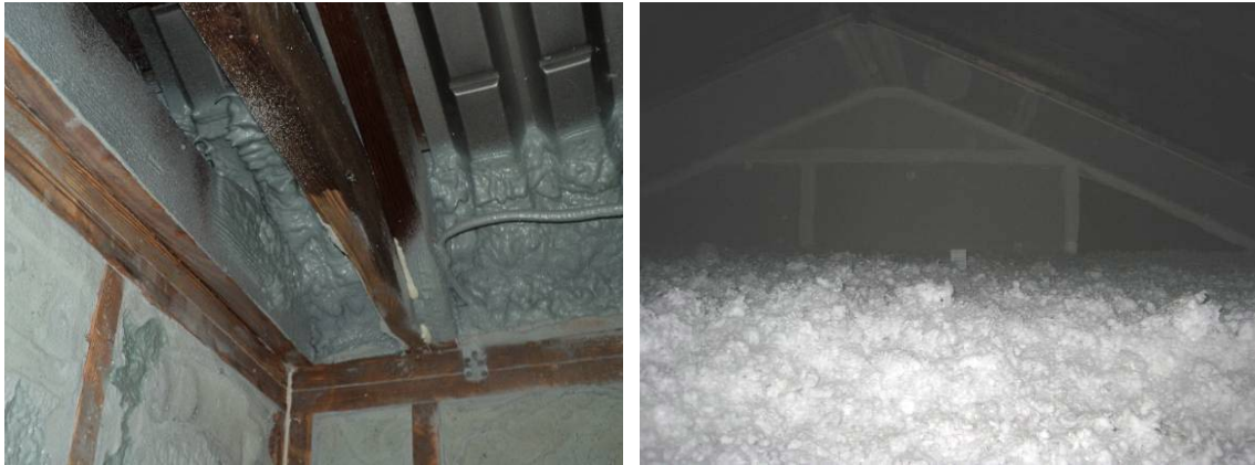
Figure 12. Baffles foamed in place and blown fiberglass in attics
