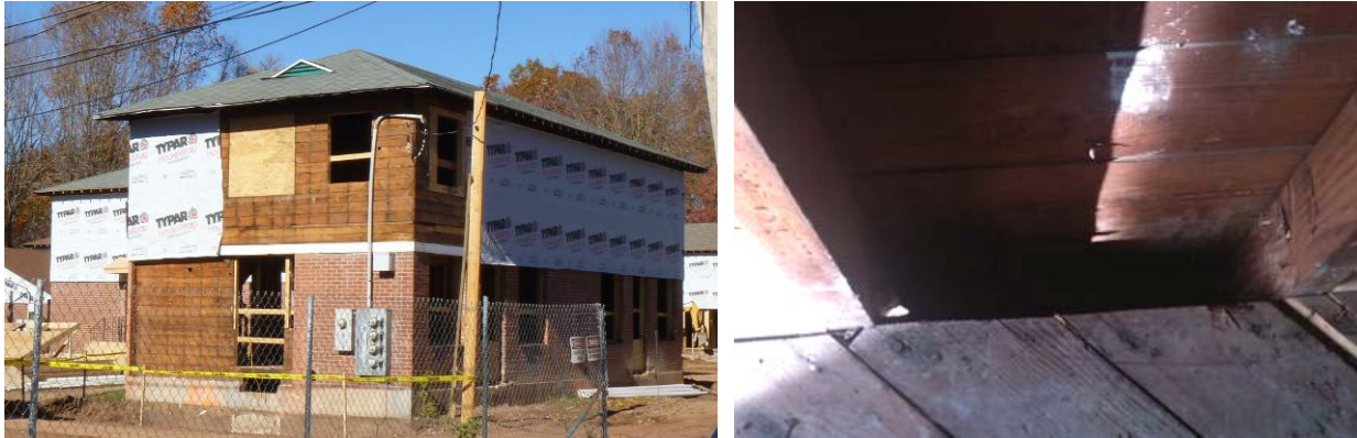
Figure 9. Above-grade wall prior to retrofit and balloon framing
