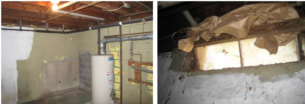
Figure 7. Basement prior to retrofit
