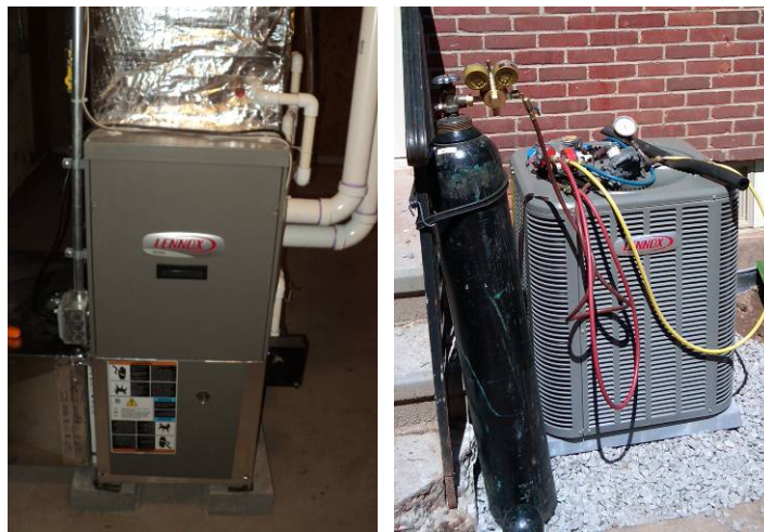
Figure 14. 94 AFUE NG condensing furnace and technician equipment for line purging
