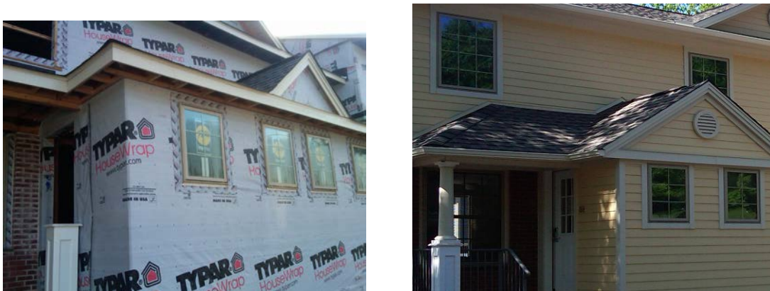
Figure 13. Windows during and after retrofit
