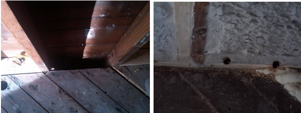
Figure 11. Balloon framing after retrofit
