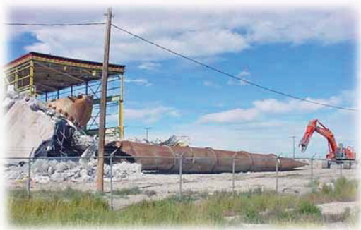
Figure 22. Demolition of the WRRTF stack.
