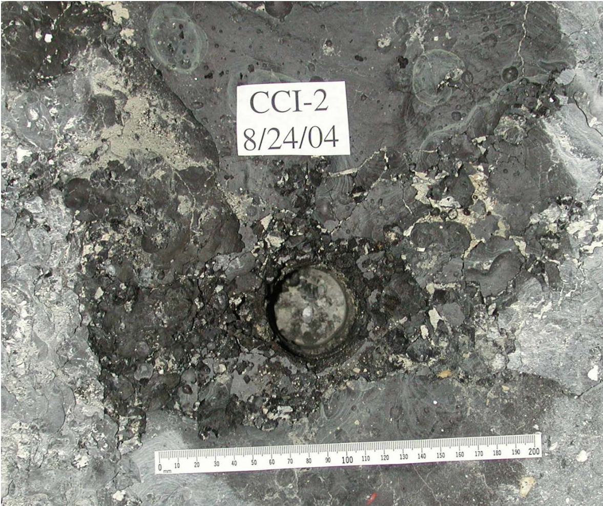
Figure 4-37. Picture of the Core Hole Drilled Near the Test Section Centerline.
