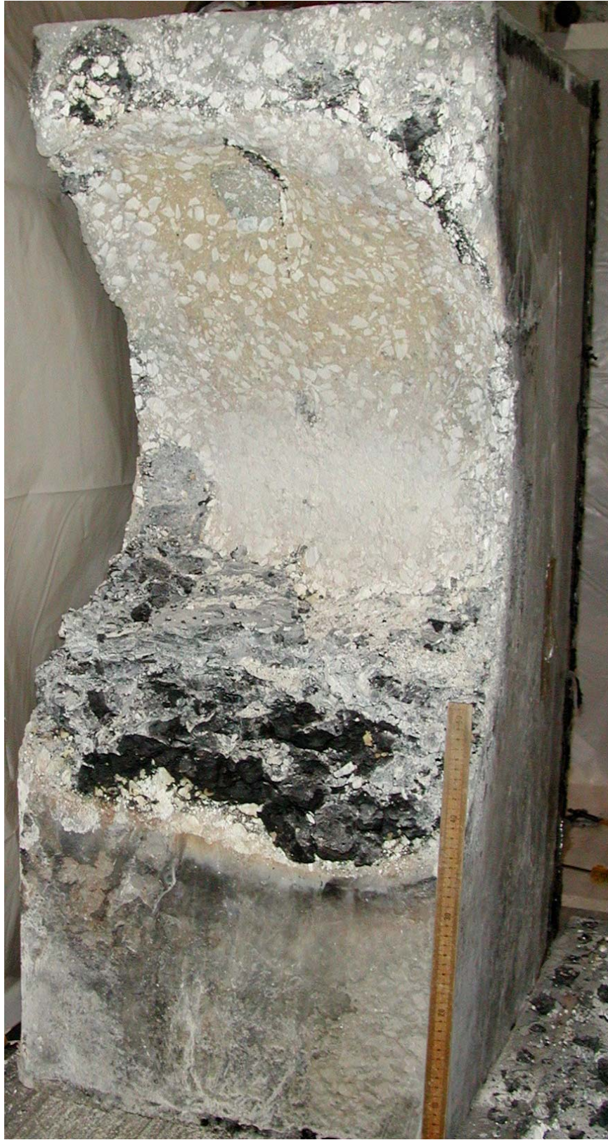
Figure 4-40. View of the South Concrete Sidewall After Removal.
