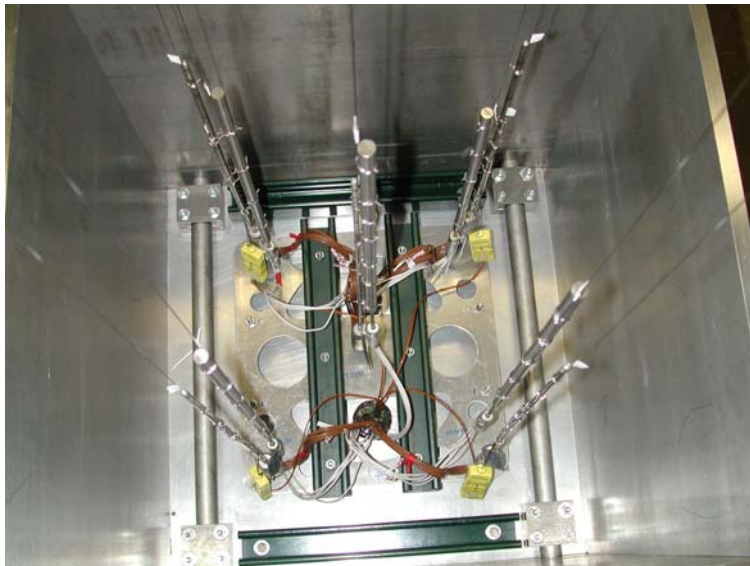
Figure 2-25. Thermocouple Arrays Installed in Basemat Concrete Form.
