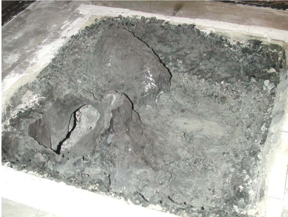
Figure 4-31. West View of Debris Top Surface After Removal of the Middle Sidewall Section.
