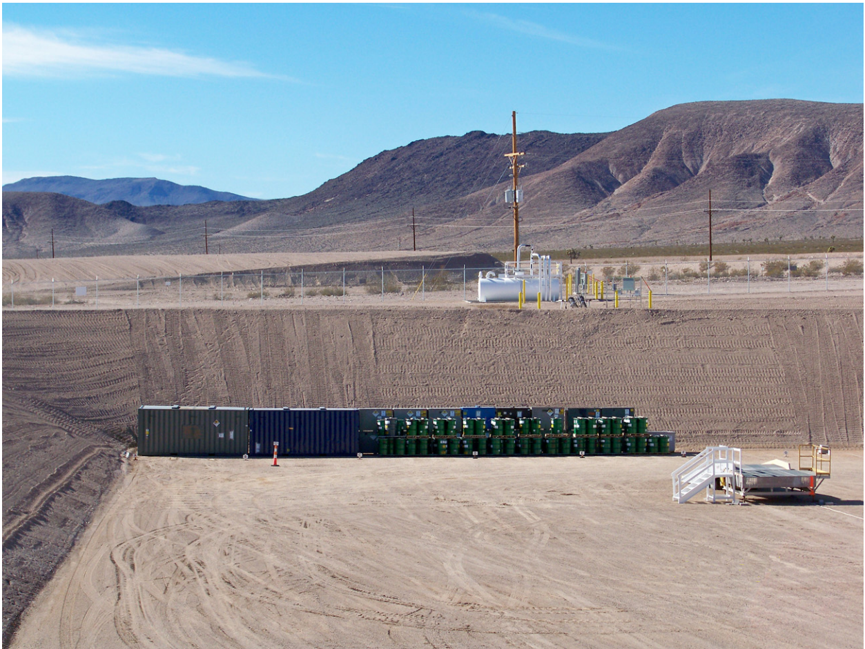
Waste Packages in Cell 18, Nevada National Security Site
