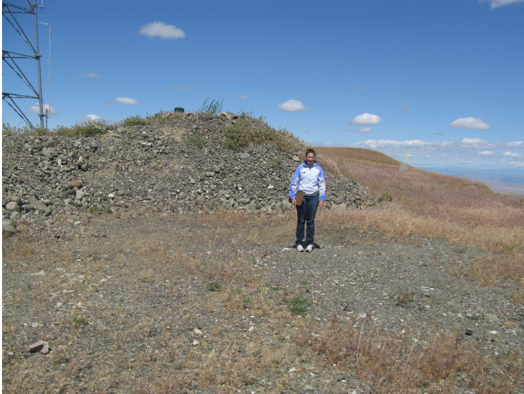
Figure B.25. Unit 4 (CCF Berms): Example of Berm Areas Sampled
