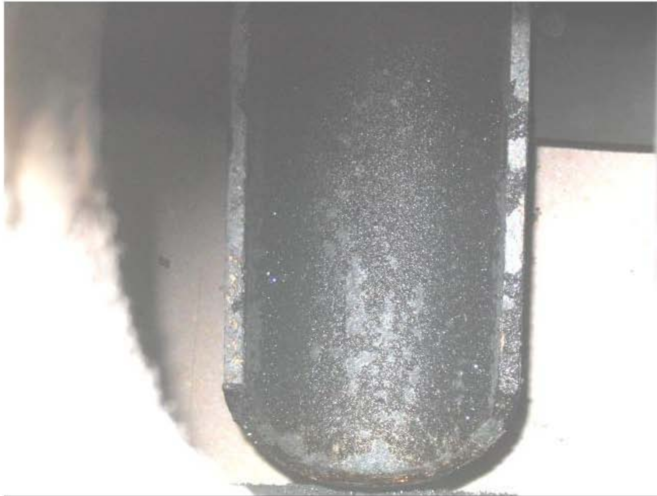
Figure 2.21. View of the bottom of the discharge trough through the view port on the south wall of the discharge chamber.
