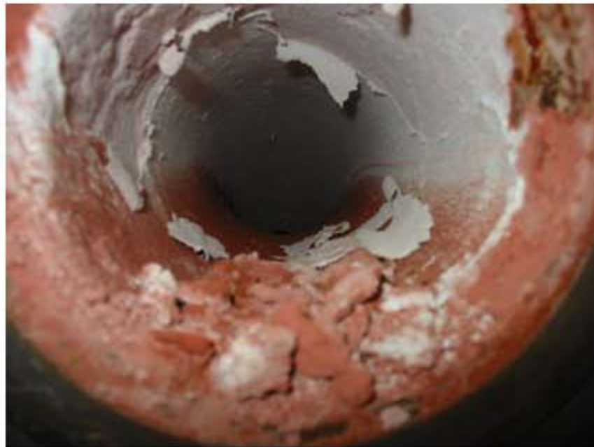
Figure 4.26. Inside view of the SBS-side of the flexible bellows (pre-cleaning) after 121.6 hours of operations during tests with LAW Sub-Envelope A1 simulants [14].
