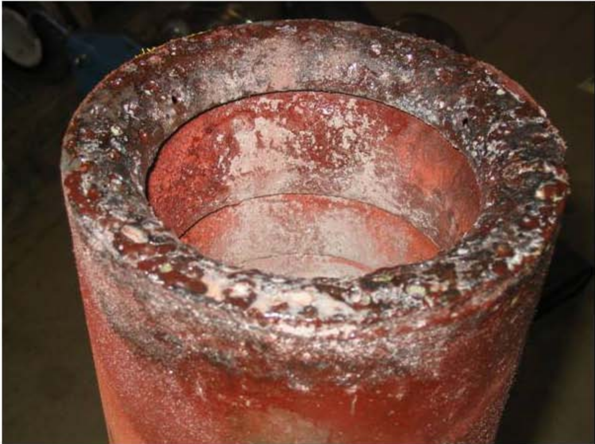
Figure 4.46. Close-up of film cooler inlet after Configuration Test 10 [30].
