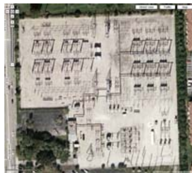
Figure 100. Flagami substation, aerial view (source: Google Maps)
