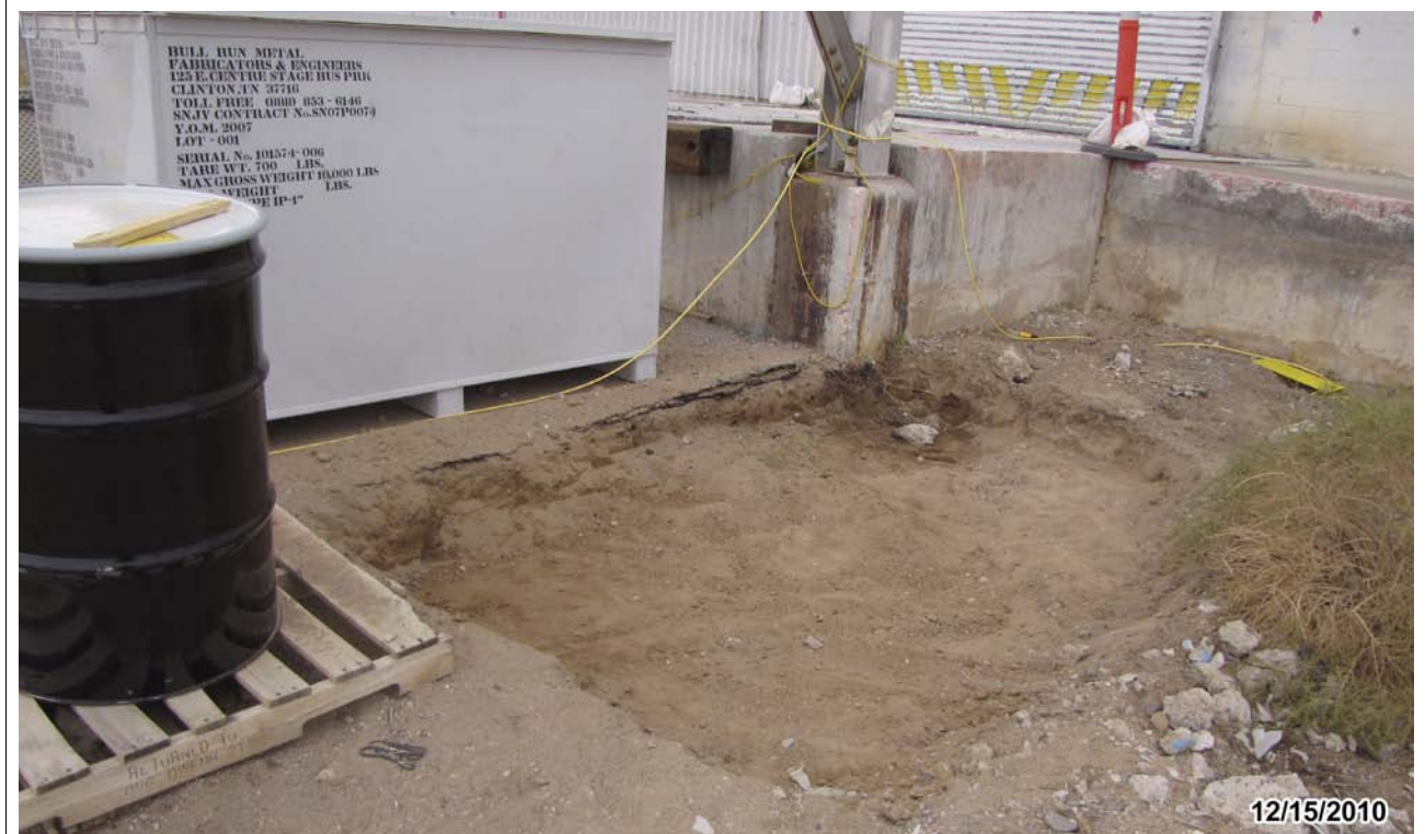
Figure 2-20 Radiological Lead-Contaminated Area
