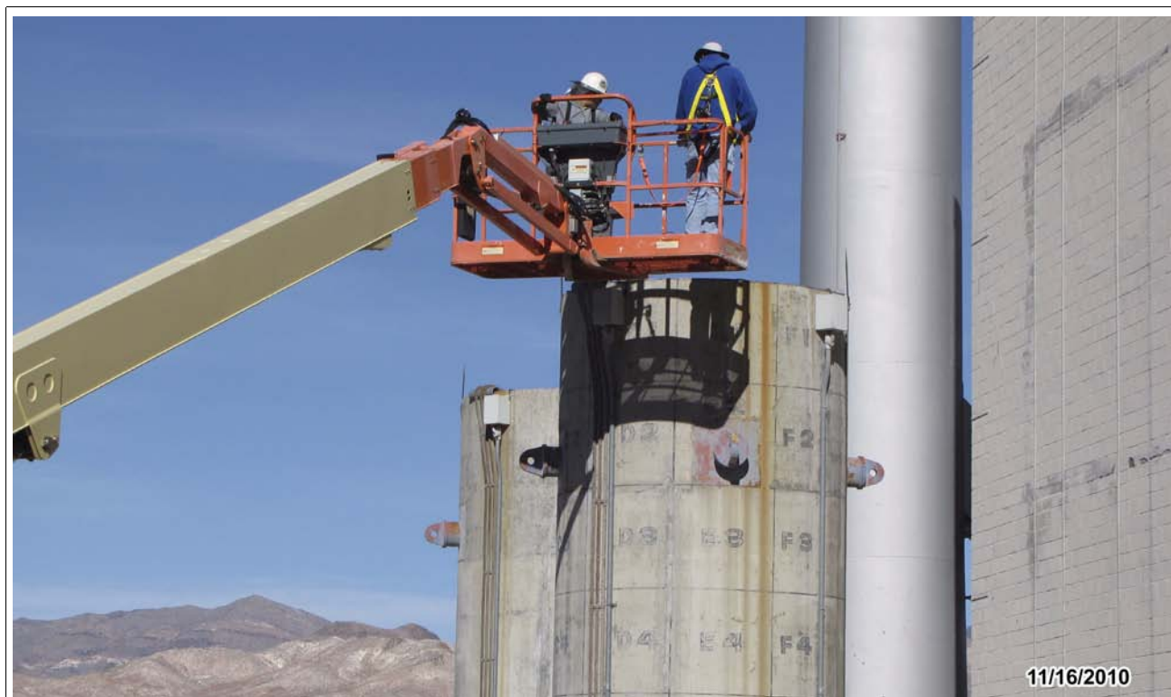
Figure 2-15 Removal of Metal Lids and Investigation of Concrete Casks
