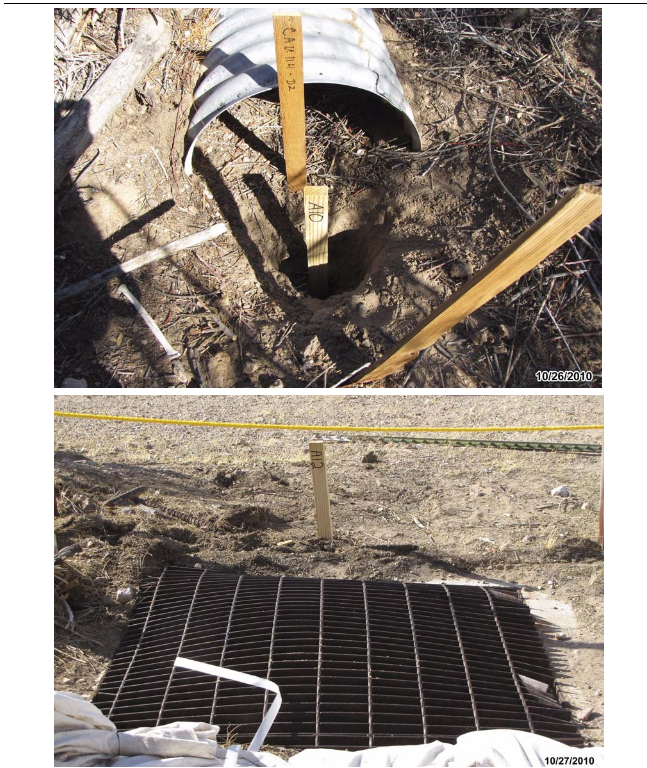
Figure 2-5 EMAD Compound Storm Drain System Outfall (top) and Catch Basin (bottom)
