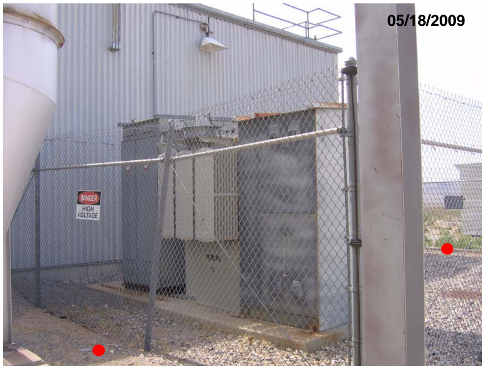
Figure B.8-4 Proposed Decision I Sampling Locations at Substations of Building 3900
