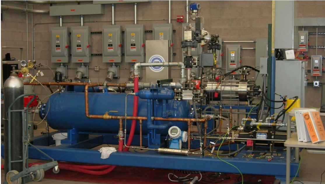
Figure 3-4: Photo of the Sandia S-CO 2 compression loop as assembled at SNL.
