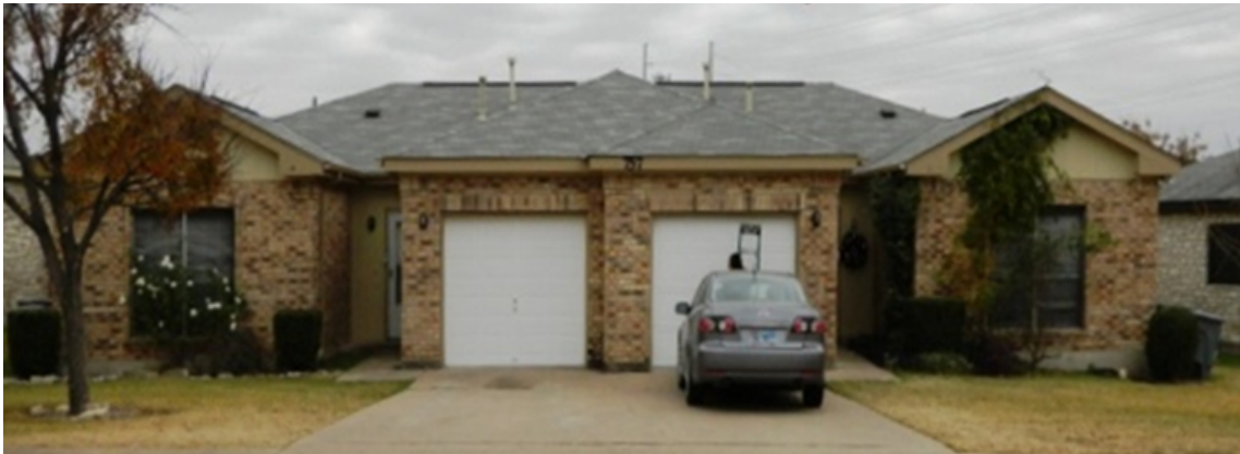
Figure 1. Austin duplex DMSHP deployment site
