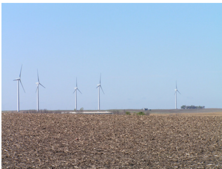
Figure 29. 8-MW Junction Hilltop Wind Project in Iowa (Photo credit: Tom Wind)
