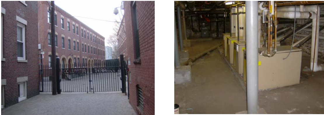
Figure 1. Exterior view of Building 3 and typical basement boiler room
