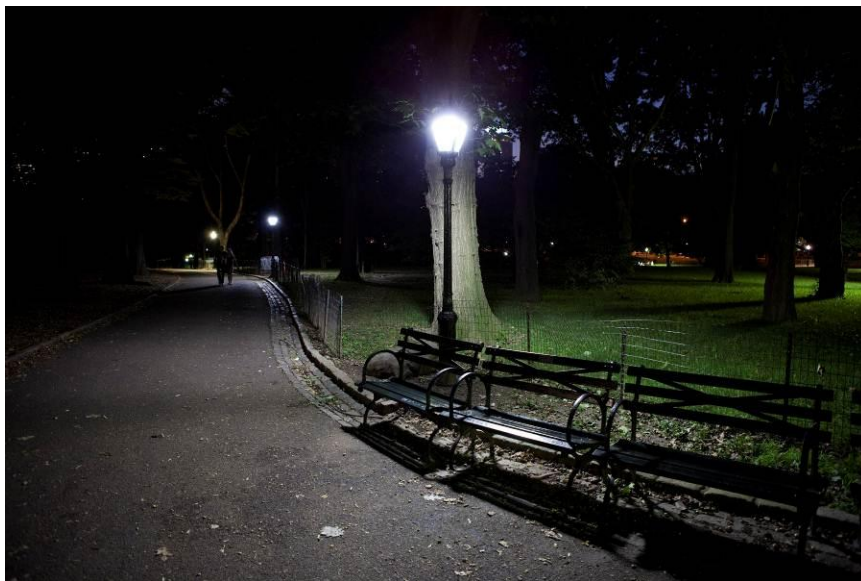
Figure 2.4. Example of symmetric distribution product (Sentry Electric) (courtesy of The Climate Group and Ryan Pyle [#70])
