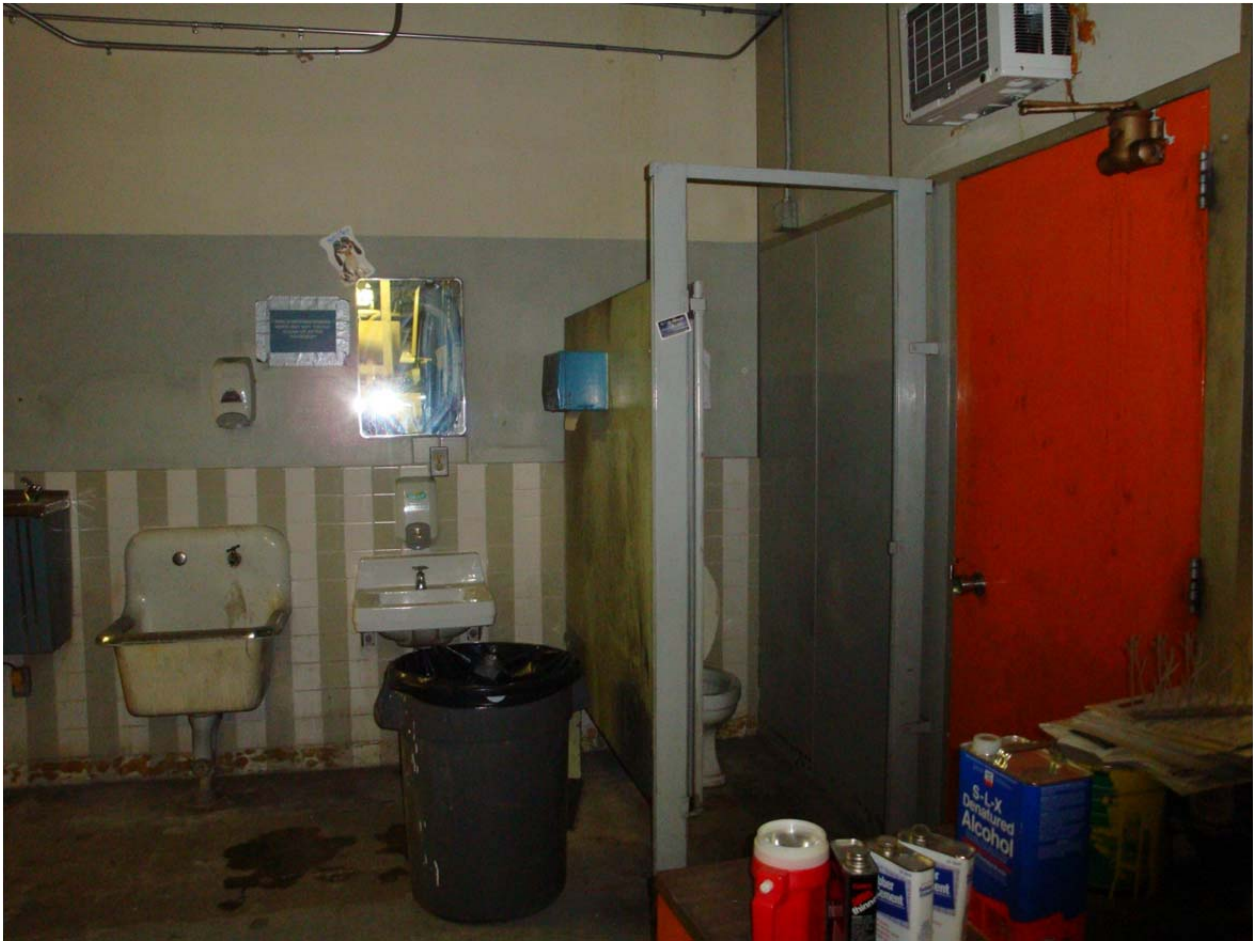
Previous central plant custodial closet and restroom
