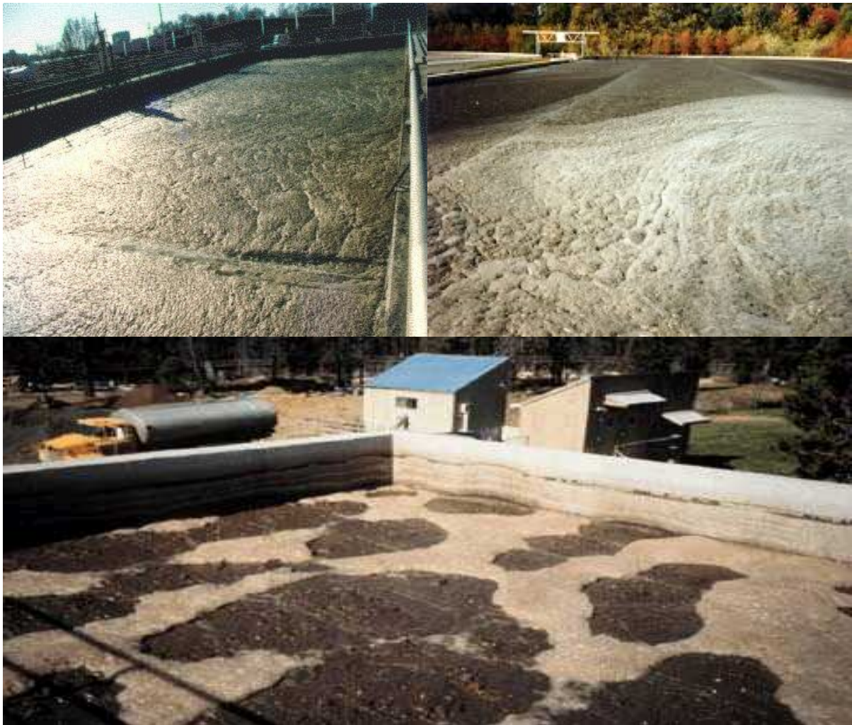
Figure 2.2 Viscous bulking causes unsettled sludge and foam in clarifiers (Retrieved from http://web.deu.edu.tr/atiksu/ana52/4ani.html , May 2015)
