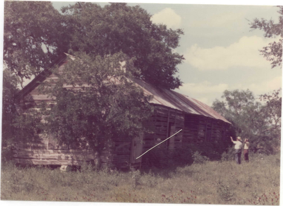
Plate 34--Claiborne Kyle's log cabin. This is probably where the Austin singers spent the night on the way to the 1853 Sängerfest in New Braunfels. Built about 1845, the structure is located near a bluff on the north side of the Blanco River, not far from the old San Antonio-Austin stagecoach road. An unusually large structure, the four-room house consists of two double-pen cabins on either side of the "dog trot" (breeze way). Except for a fallen east chimney the building is remarkably well preserved. The location of the property, now owned by Tom Arch Allen of Kyle, is about three miles southwest of Kyle.
