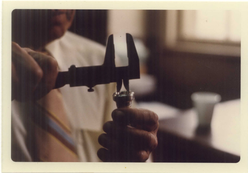
Fig. 7--Measuring the inside cup diameter
