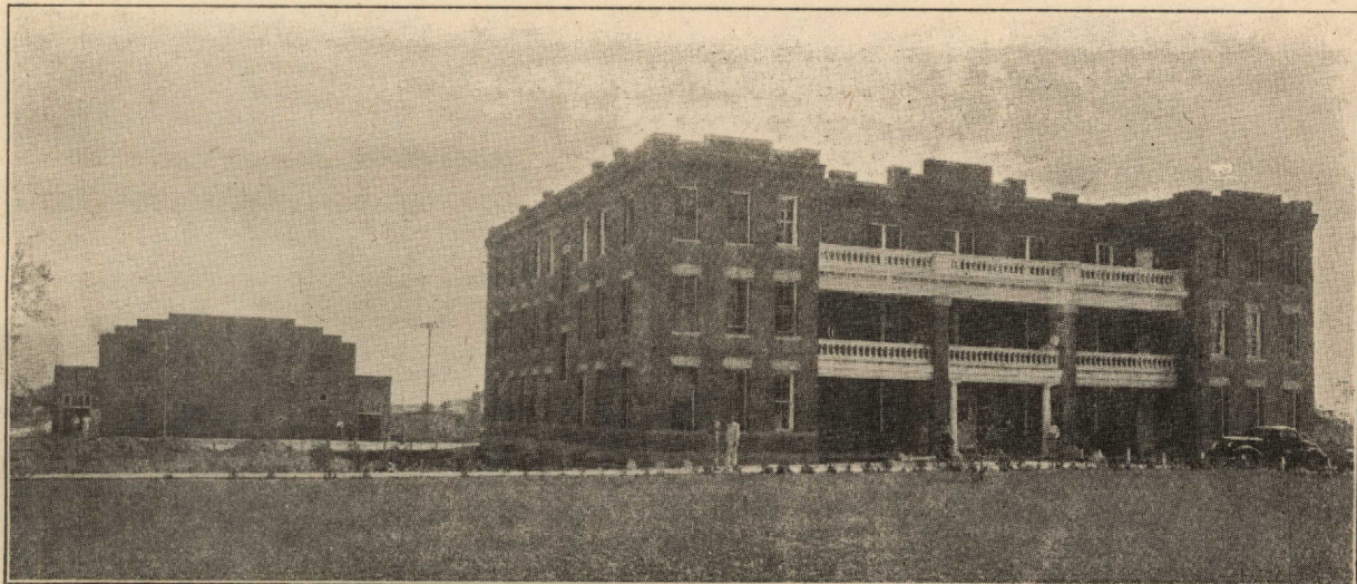
Boys' Dormitory With Gymnasium in the Background Decatur Baptist College
