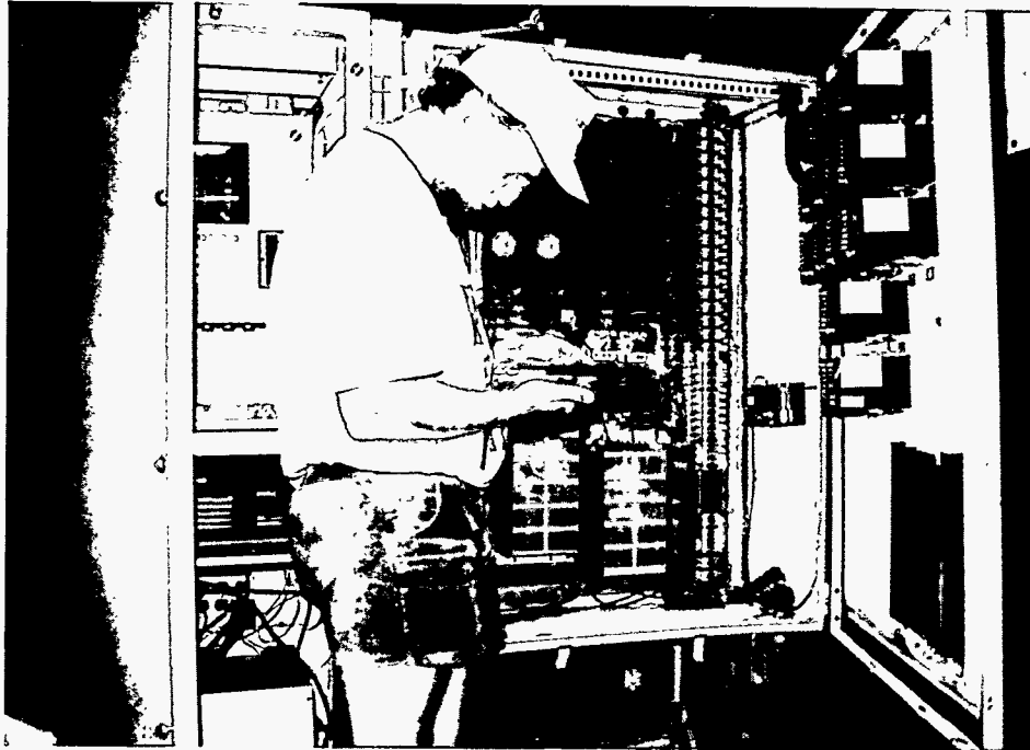
Fig. 4.9. At the Kwajalein data collection system, an I&C engineer checks the current load on the roots blower used to inject air into the wells.
