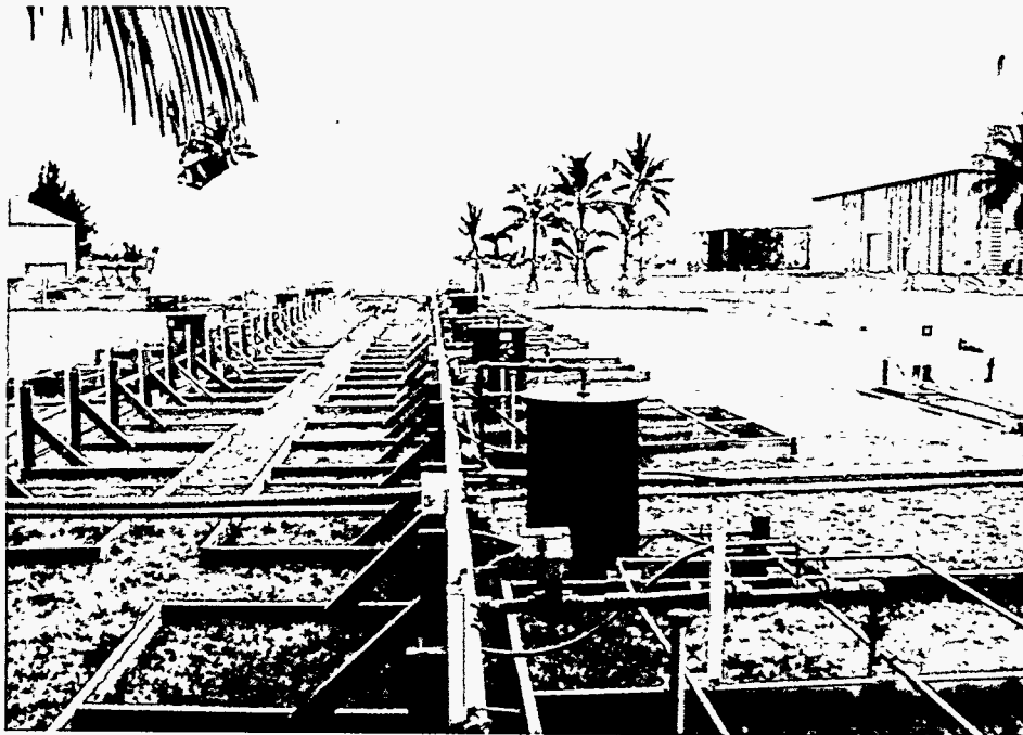
Fig. 4.10. A view of the Kwajalein air injection and water distribution systems for many wells.
