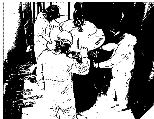
▲ FIGURE 7. The TMRS insert being placed into the target crypt.
