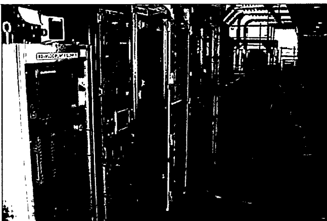
▲ FIGURE 15. The SCR power supply and klystron electronics control racks.
