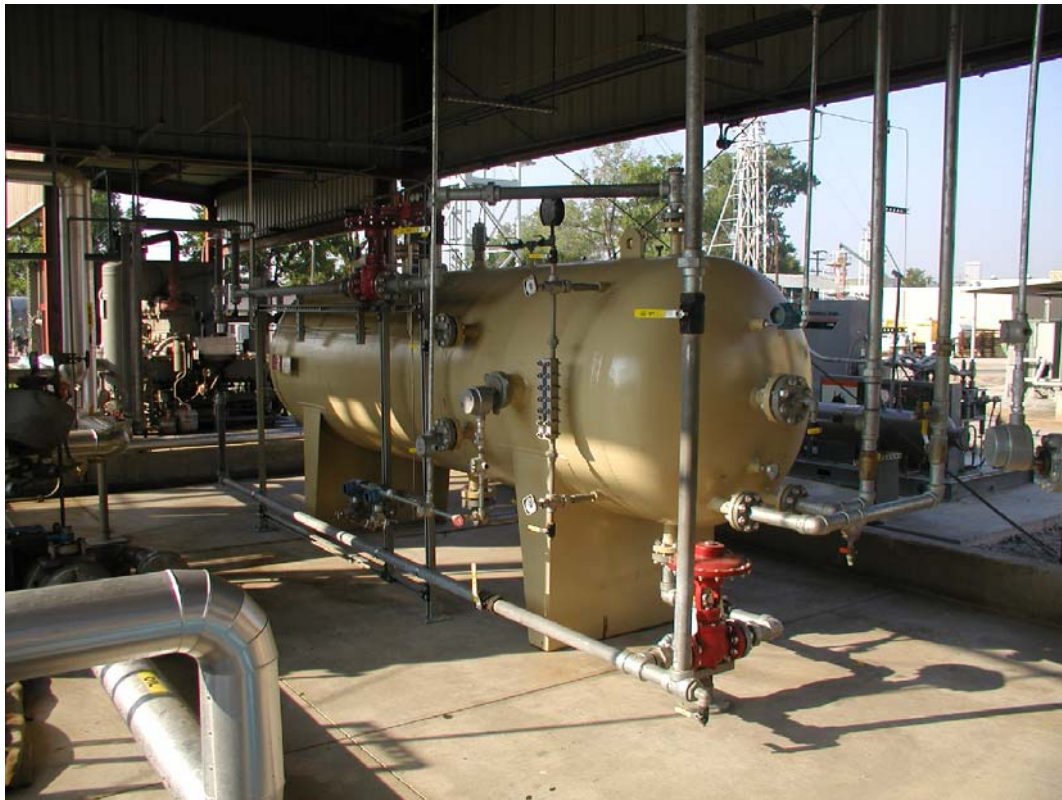
Figure 2.11 – Construction of Water System
