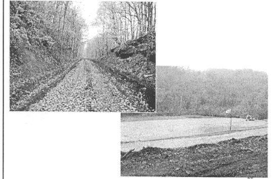
South Well Site, April 2003
