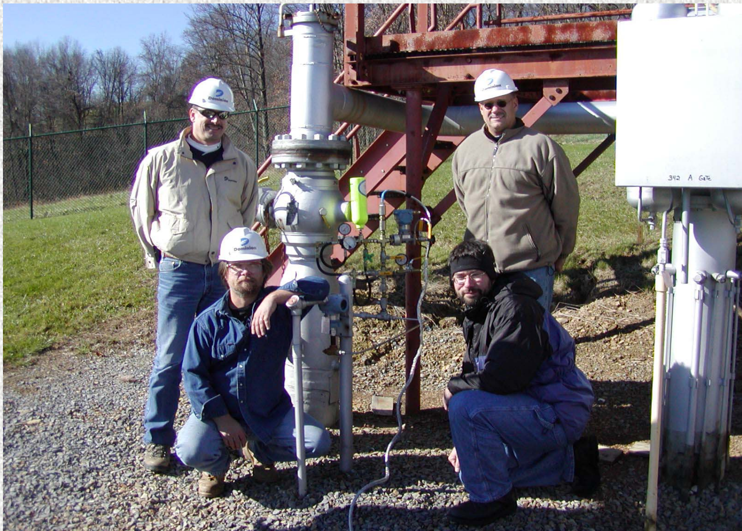
Figure 10 - Dominion Transmission Inc. 900-psi 24-inch transmission line access near Waynesburg, PA. Engineers Jim Parsons, Bill Ruffner, John Hart and WVU research assistant Richard Guiler next to the “Portable Acoustic Monitoring Package” (PAMP).
