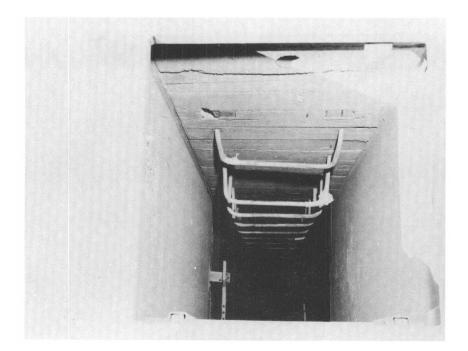
Fig. 3.68—Emergency-exit shaft (structure CAa). Note bent climing rungs and straightened hinge strap.
