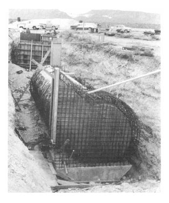
Fig. A.15—Interior formwork erected (structure CA) (May 22, 1957).
