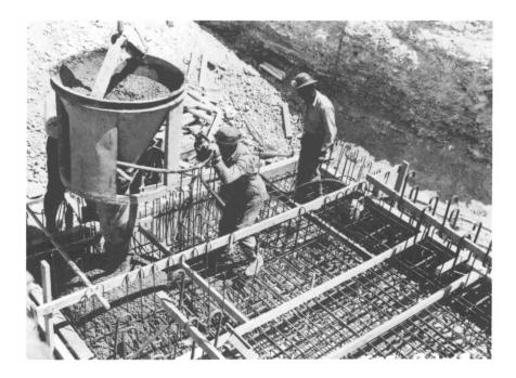
Fig. A.4-Base-slab concrete placement (structure RA) (Apr. 29, 1957).
