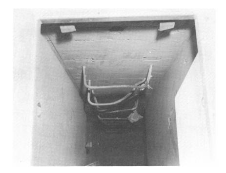
Fig. 3.79—Emergency-exit shaft (structure CAb). Note bent climbing rungs and straightened hinge straps.
