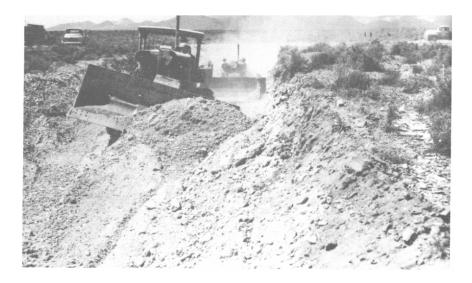
Fig. A.24—Use of blade rippers during excavation.
