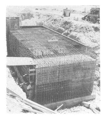
Fig. A.9—Wall- and roof-slab reinforcement placed; erecting exterior formwork (structure RA) (May 10, 1957).
