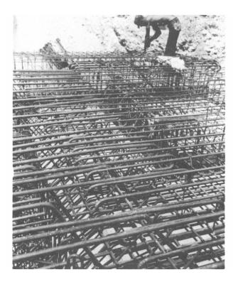
Fig. A.8—Detail of roof-slab reinforcement (structure RA) (May 8, 1957).
