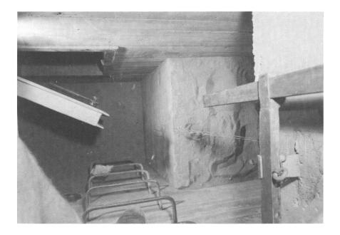
Fig. 1.18—Emergency exit blast door (structure CA).
