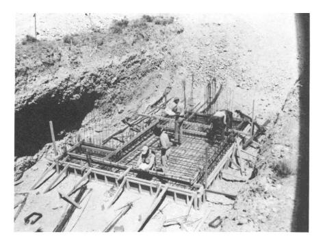
Fig. A.19-Placement of base-slab reinforcement (structure RC) (May 1, 1957).
