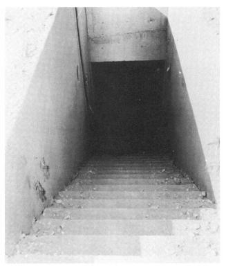
Fig. 3.47—Looking down entrance facing away from GZ, showing cracks between parapet wall and interior and exterior walls (structure RAc).
