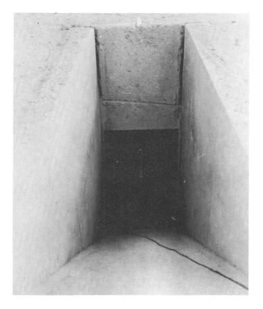
Fig. 3.50—Looking down entrance toward GZ, showing separation of parapet wall from interior and exterior walls and bowing of ramp wall (structure RAc).
