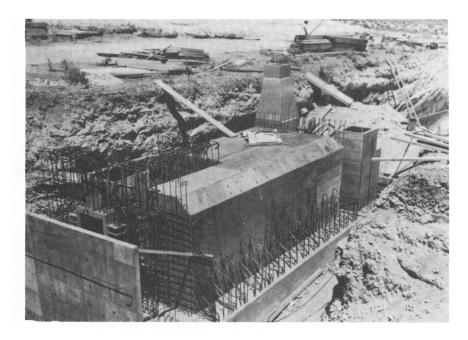
Fig. A.6—Interior formwork erected; placement of wall reinforcement begun (structure RA) (May 3, 1957).
