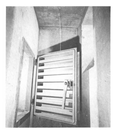
Fig. 1.26 --- Emergency-exit blast door (structure RC).
