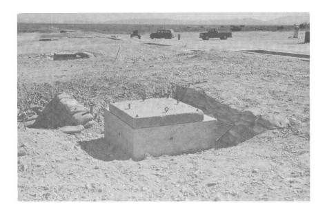
Fig. 1.12—Above-ground section of vent stack (structure RA).
