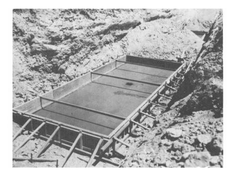
Fig. A.2—Sub-base concrete placement completed (structure RA) (Apr. 27, 1959).
