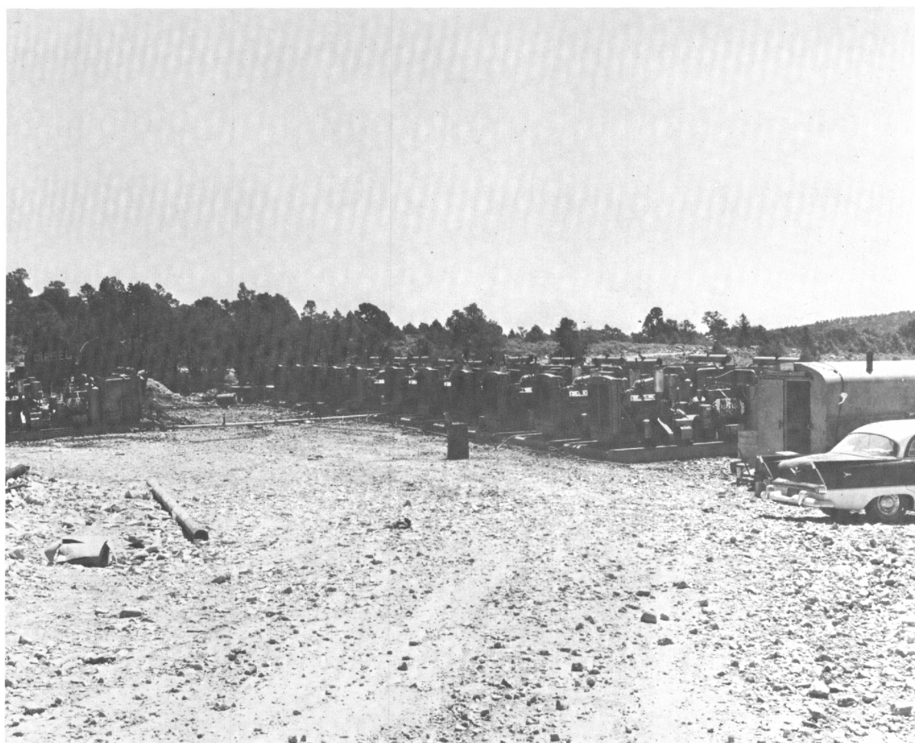
Fig. 16. View of a bank of air compressors being used as the air supply for direct air circulation on a 64" diameter hole. Photo-USAEC.
