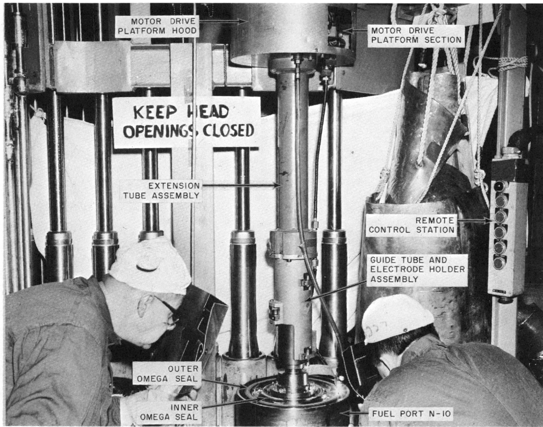
Figure 17a. Welding the Outer Omega Seal on Fuel Port N-10.
