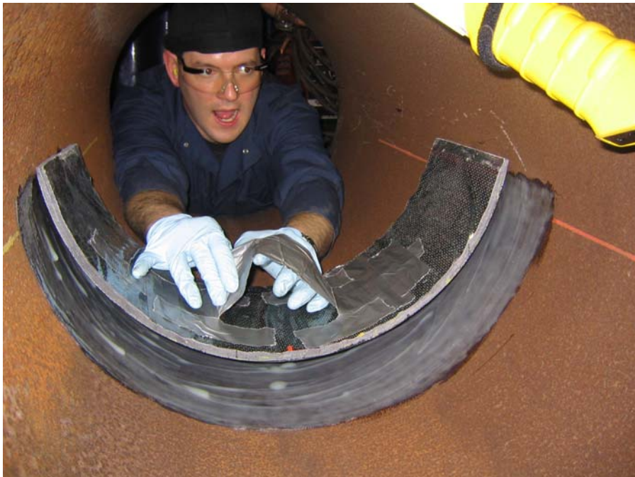
Figure 25 - Installation of Repair Patch
