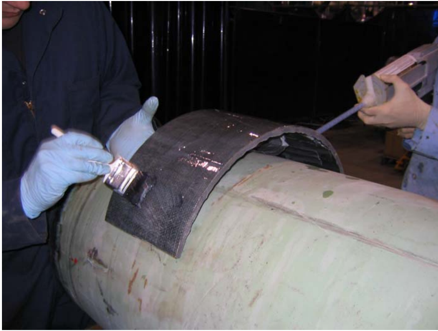
Figure 24 - Application of Adhesive to Repair Patch
