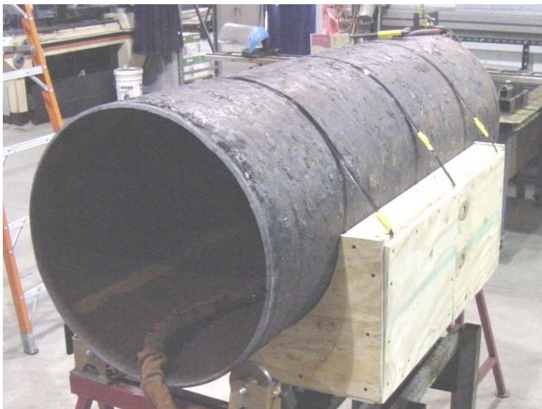
Figure 44 - Orientation of Pipe Section with Dirt Box for Weld Deposition Repair
