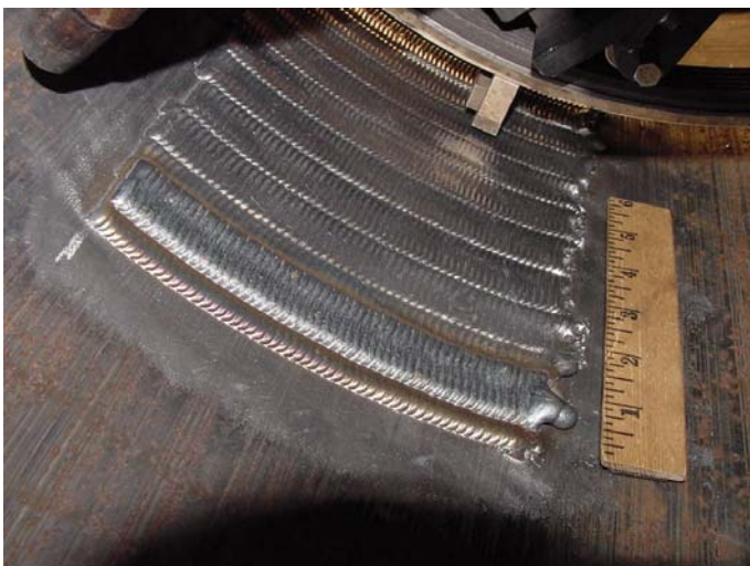
Figure 50 - First Pass of Second Layer of Deposited Weld Metal on Inside Pipe Diameter
