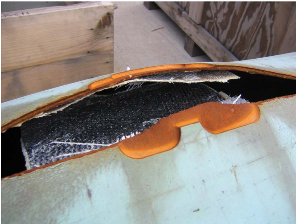
Figure 92 - Failure Initiation Site For Burst Tested Pipe With Carbon Fiber-Reinforced Liner Repair
