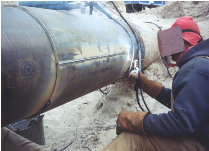
Figure 1 - Installation of a Full-Encirclement Repair Sleeve
