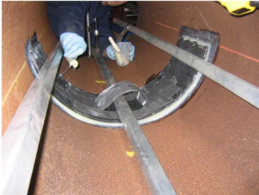
Figure 26 - Clamping Bars Used to Hold Repair Patch in Place
