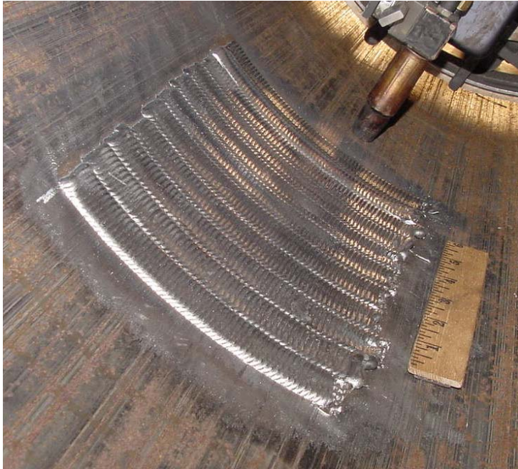
Figure 49 - Finished First Layer of Deposited Weld Metal on Inside Pipe Diameter
