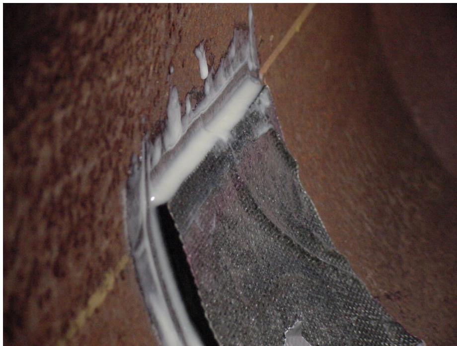
Figure 27 - Adhesive Fillet Around Repair Patch
