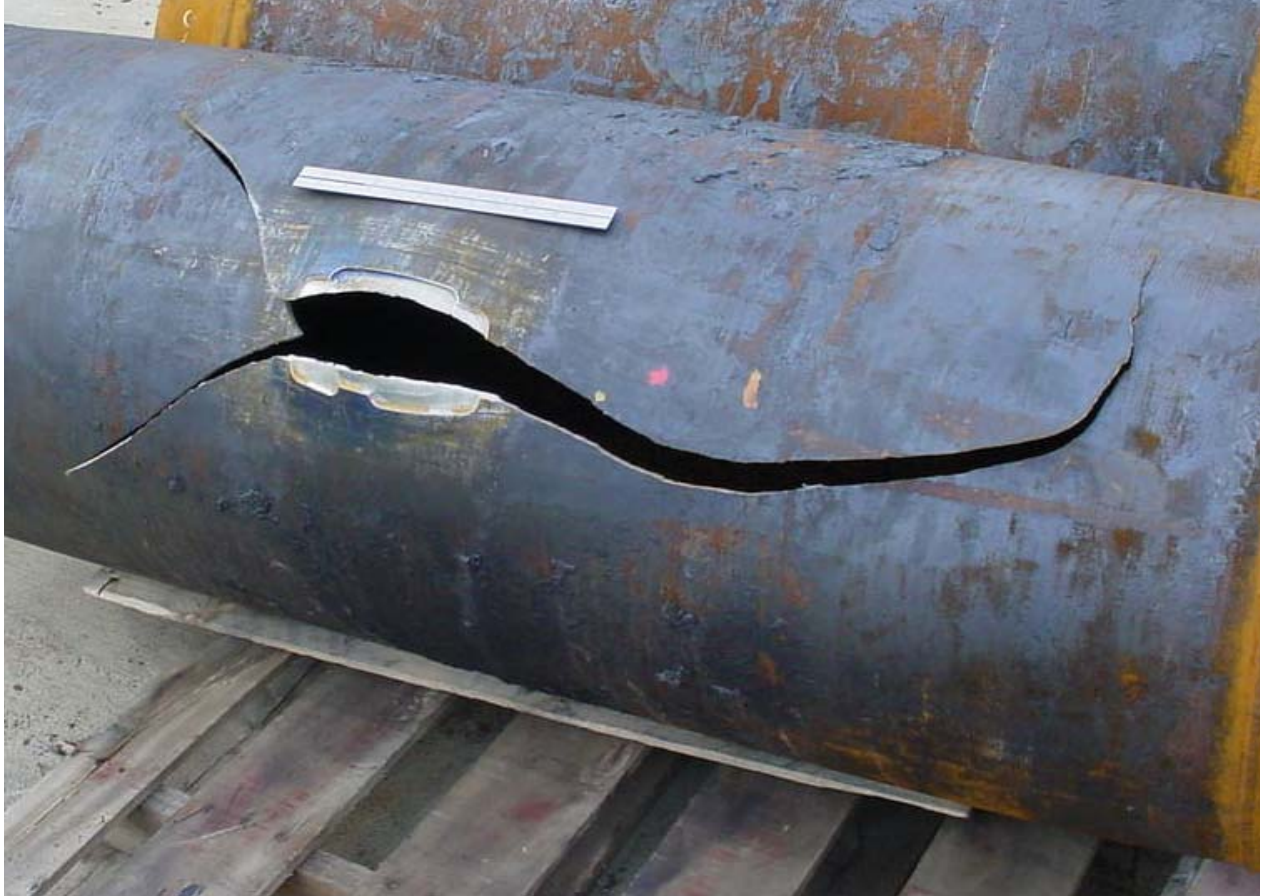
Figure 117 - Hydrostatic Burst Specimen of 558.8 mm (22 in.) With Un-Repaired Damage
