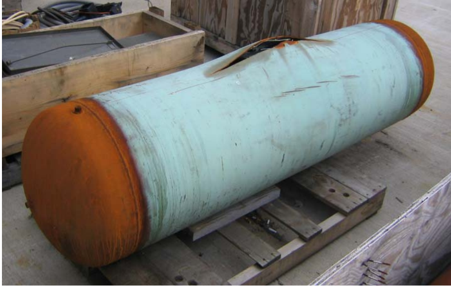
Figure 91 - Pipe With Carbon Fiber-Reinforced Liner Repair After Burst Test
