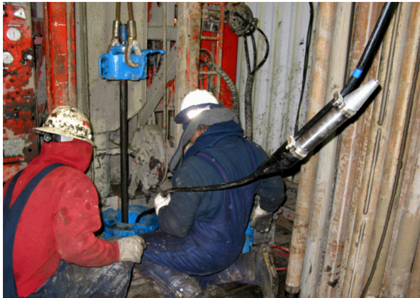
Figure 2. Deploying VSP Receiver Array into the Wellbore
