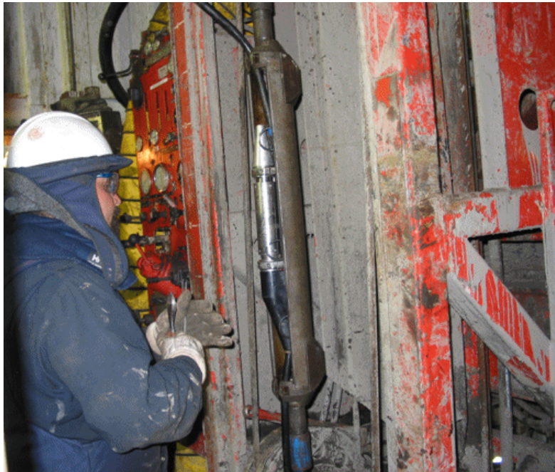
Figure 6. Installing Receiver into Pod
