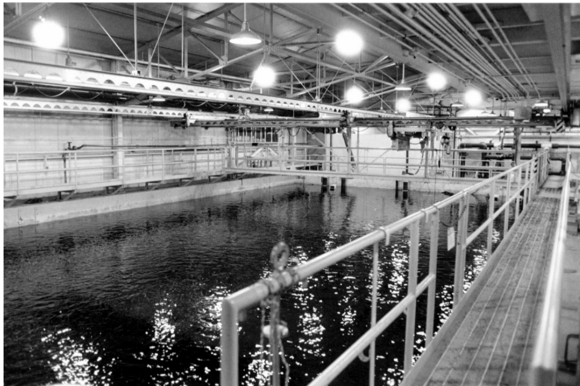
Figure 1. CPP-603 fuel storage pools contain significant amounts of sludge in the bottom.
