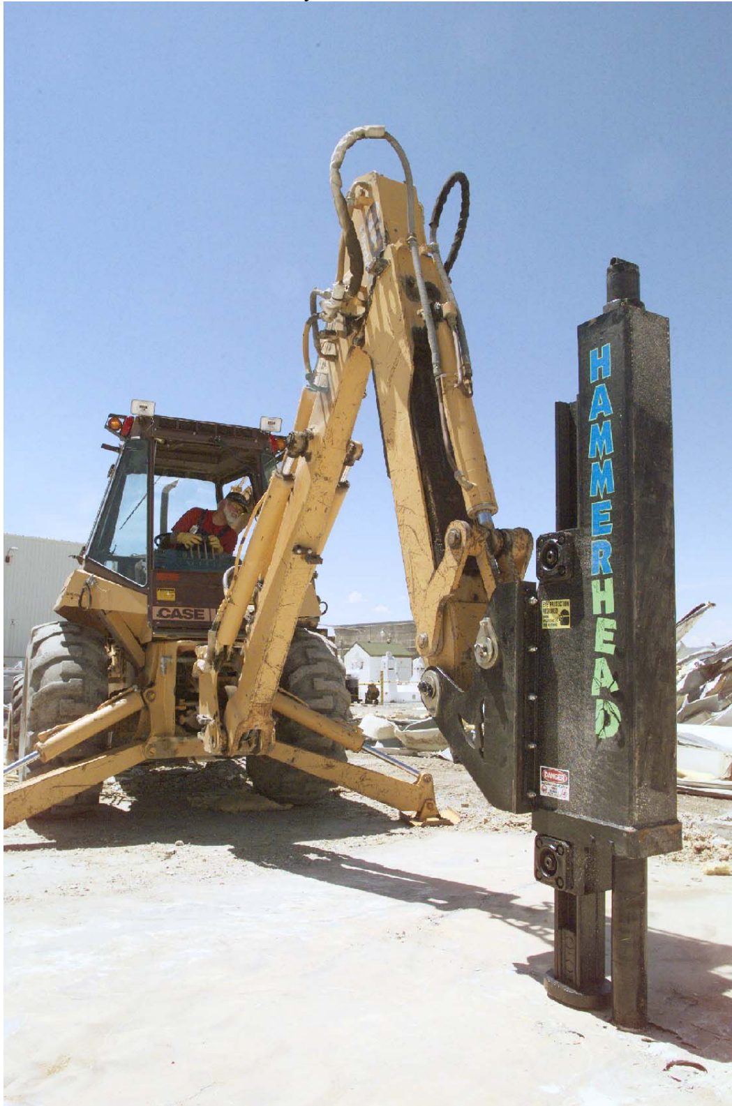
Figure 3. The Hammerhead reduced rock-fly and dust generation during pad demolition.
