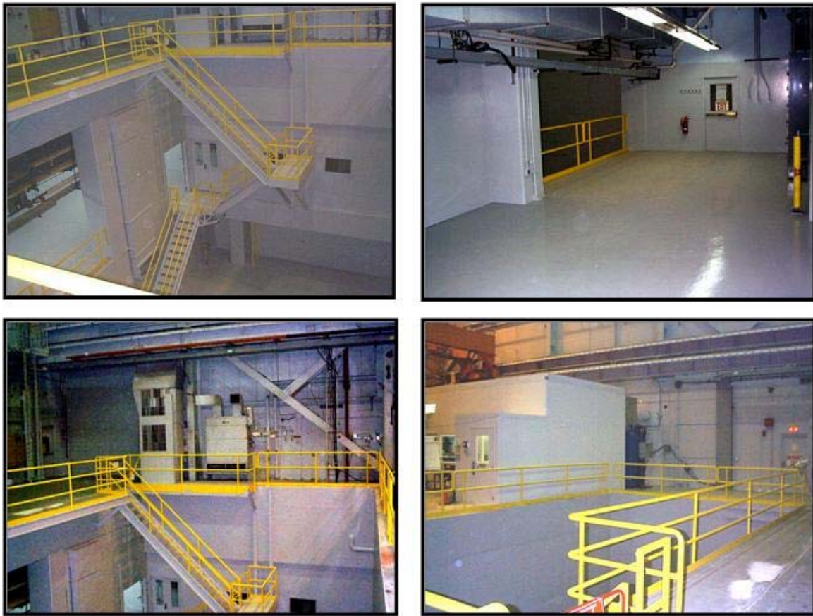
Fig. 4. Building 7602 Final Conditions.
