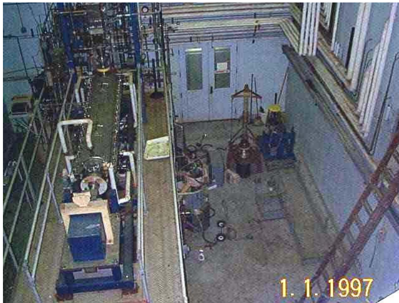
Fig. 1. View of Digester Pit Prior to Remediation
