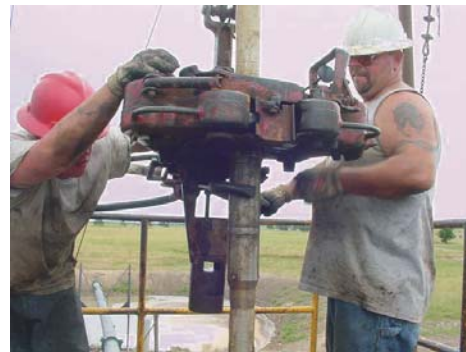
Short Radius Composite Drill Pipe being added to the drill string.
