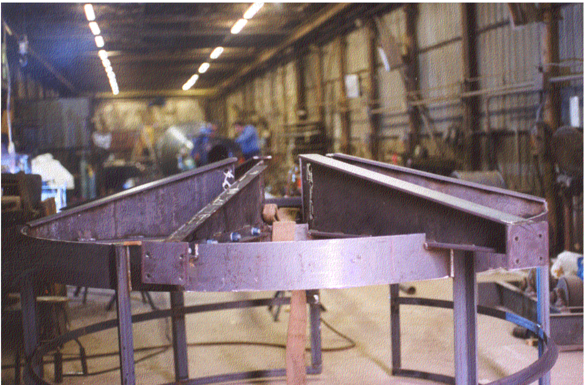
Figure 3.4 - Fabrication of One of Five Personnel Access Platforms
