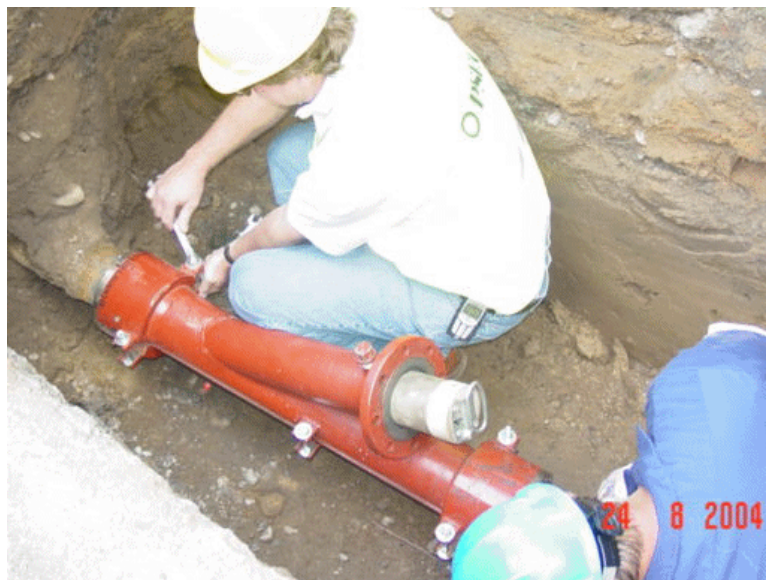
Figure 40. Attaching Entry Fitting to Pipe Prior to Welding
