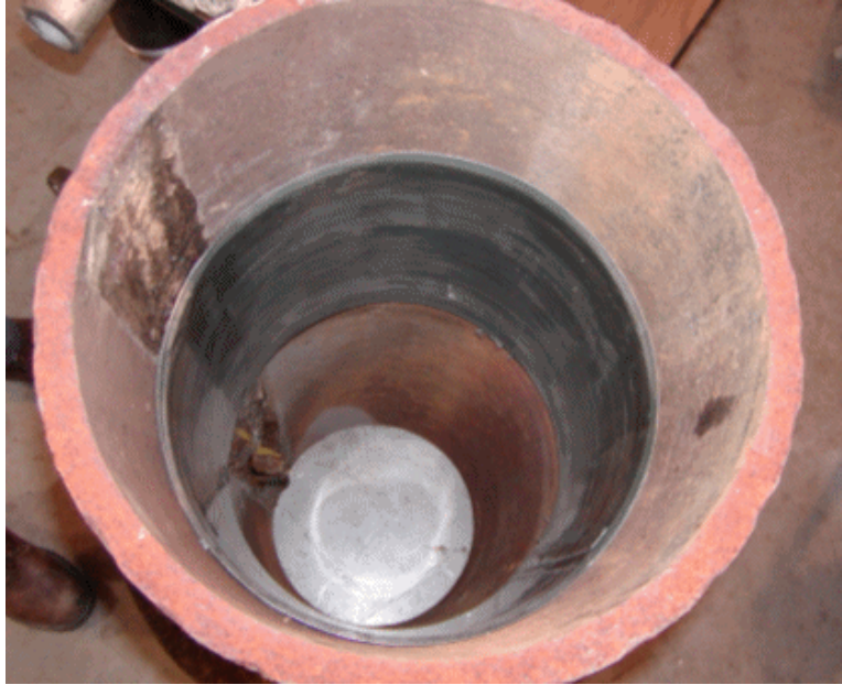
Figure 11. Successfully Installed Repair Sleeve
