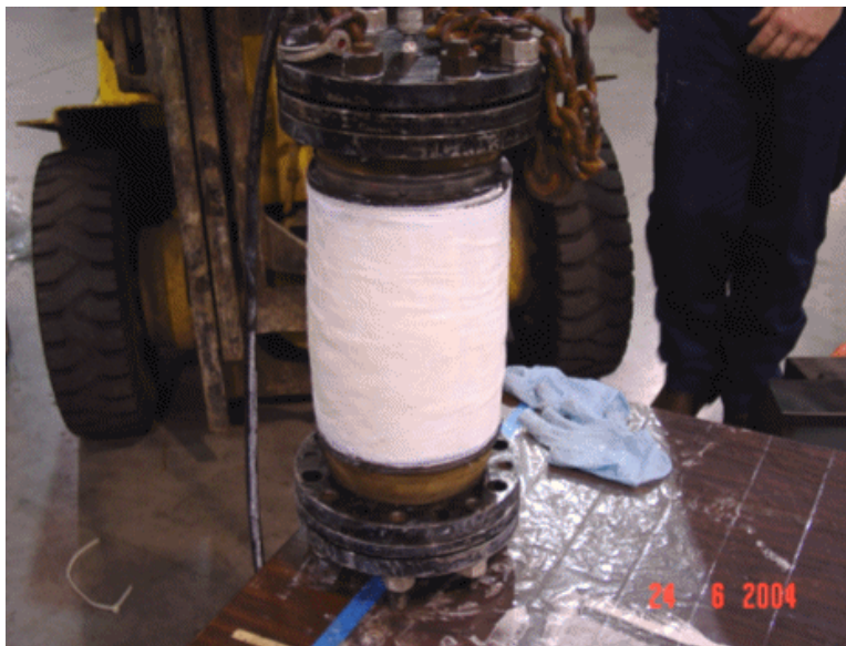
Figure 8. Repair Sleeve with Epoxy Applied
