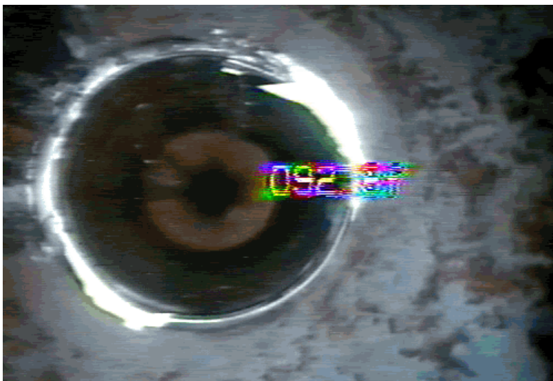
Figure 43. Successfully Set Patch at 93.7 ft
