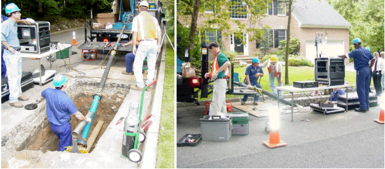
Figure 39. Field Test Site
