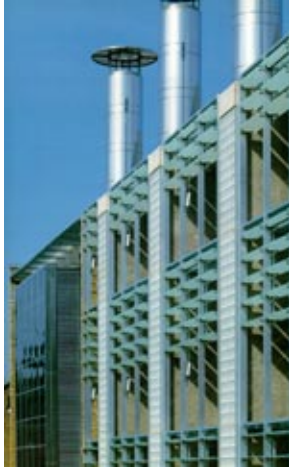
Automated translucent glass louvers at the Environmental Building, Building Research Establishment, Garston, UK (see detailed case study).
