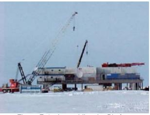
Figure E-4. Assembling the Platform
