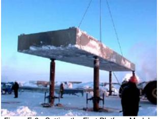
Figure E-3. Setting the First Platform Module
