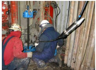
Figure E-10. Deploying VSP Array into Well
