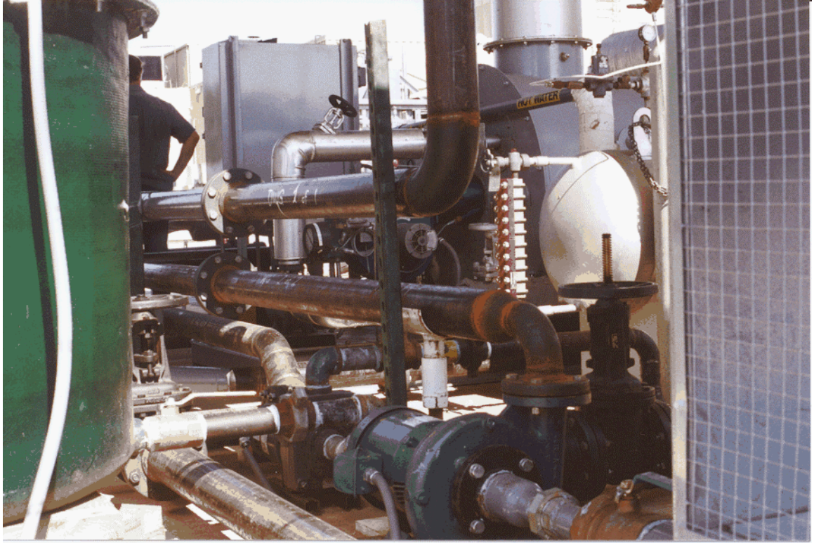
Figure 3.5- Suction Piping
