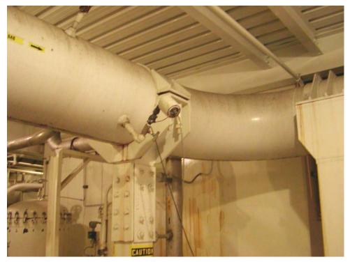
Figure 4-8. Heated Pressure Sensor (Suction Lateral); Dresser-Rand TCVC10; Dominion Groveport Station Unit 1; April 20, 2005
