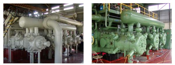
Figure 1-1. TLA6 (2,000 HP) and GMW10 (2,500 HP) in Pipeline Service
