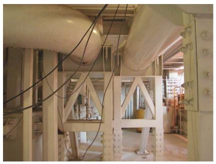
Figure 4-6. Bracing on Lateral Lines; Dresser-Rand TCVC10; Dominion Groveport Station Unit 1; April 20, 2005
