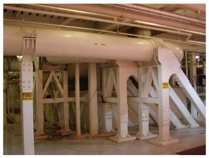
Figure 4-5. Bracing on Lateral Lines; Dresser-Rand TCVC10; Dominion Groveport Station Unit 1; April 20, 2005
