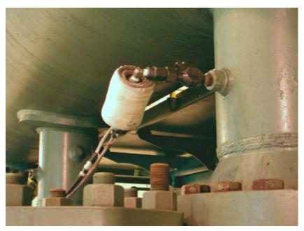
Figure 4-4. Heated Pressure Sensor Installed on Suction Nozzle; Dresser-Rand TCVC10; Dominion Groveport Station Unit 1; April 20, 2005
