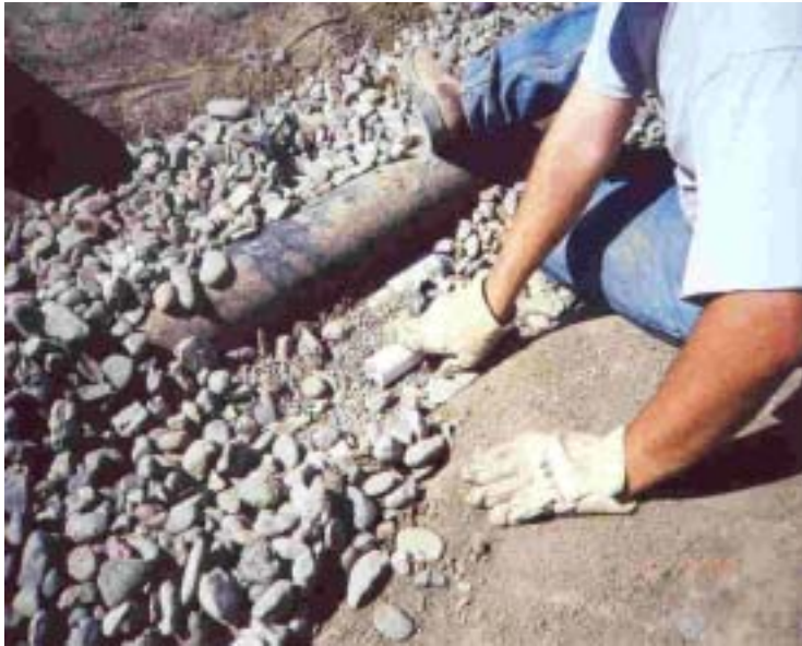
Image 6-2: Pressure tubes installed in LCRS trench
