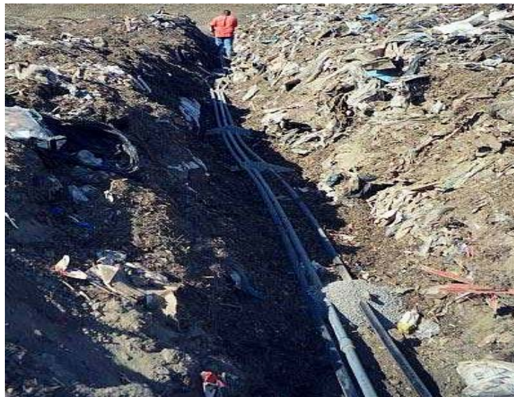
Image 5-2: Leachate injection laterals in trench
