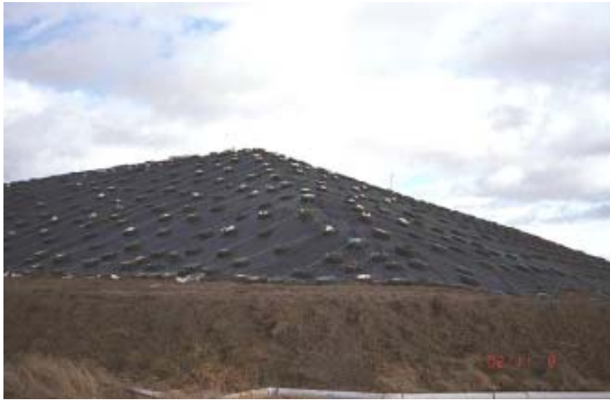
Image 4-2: West-side anaerobic cell surface liner.
