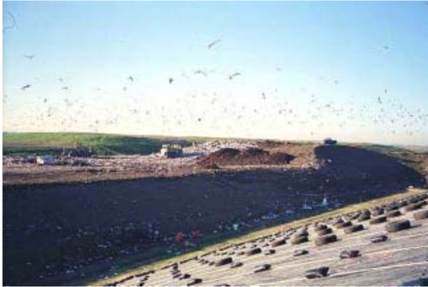
Image 4-1: Waste placement in the west-side cell
