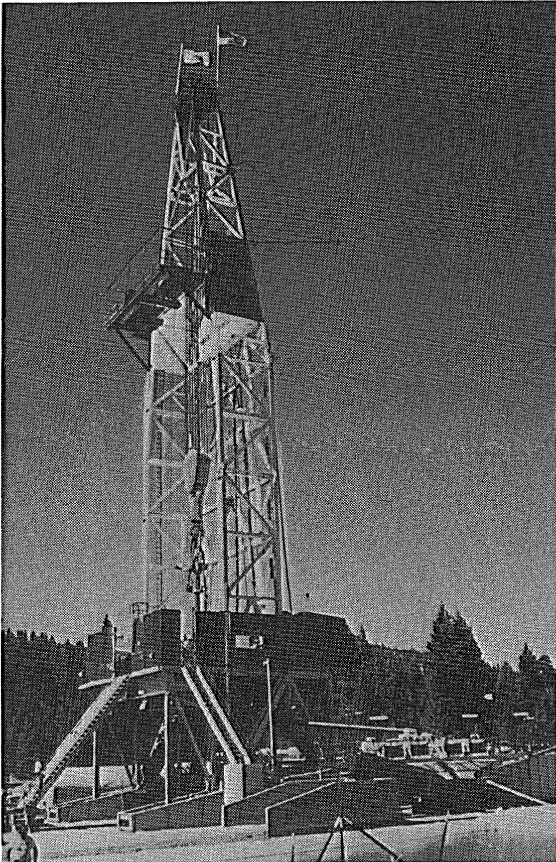
FIGURE 20 DRILLING RIG AT LONG VALLEY SITE
