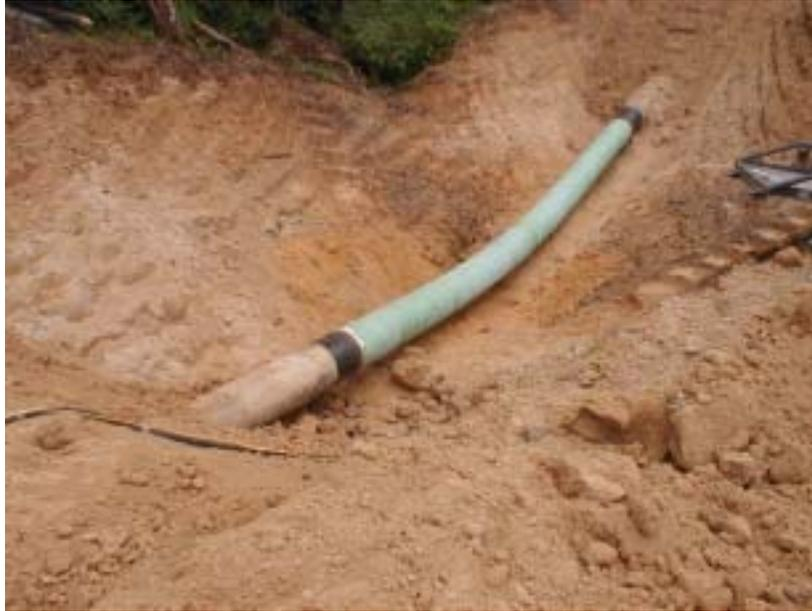
**Figure 34. Photograph of replacement pipe before burying**
