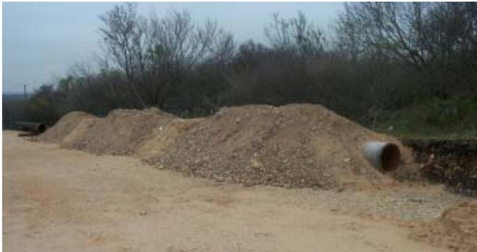
**Figure 17. Photograph of the 24.4 m (80-foot)-long, 610-mm (24-inch)-diameter pipe buried under approximately 0.6 m (2 feet) of soil**
