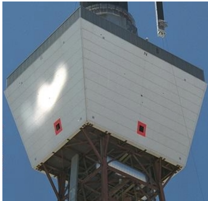
Figure 2-3. Solar Two heliostat beam tracking the BCS target.
