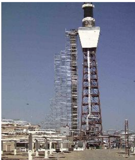
Figure 4-6. Chute on one side of the tower in which the nitrate salt was prilled for removal from the site.
