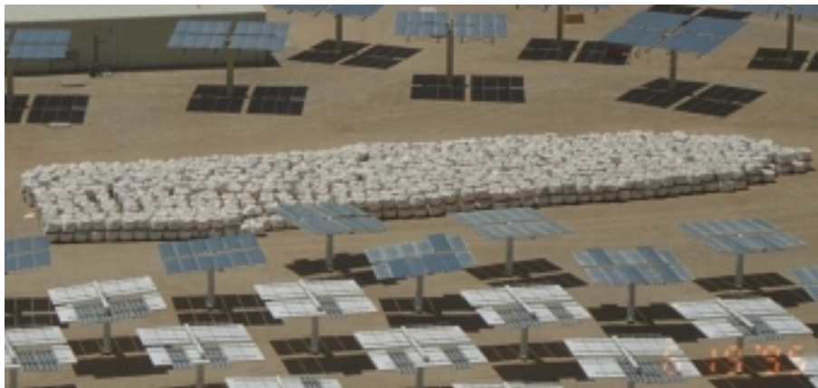
Figure 4-3. 1380 tonnes of nitrate salt awaiting melting at Solar Two.
